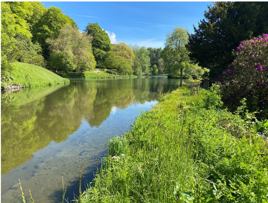
Figure 3-1: View along Garden Lake Embankment Crest
