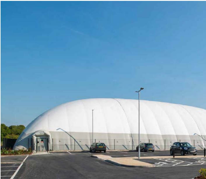
Fig. 24 External of typical airdome
