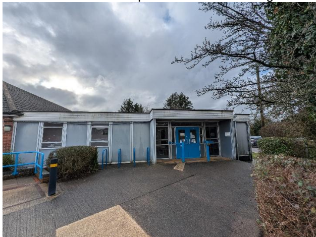
Plate 2: Northwestern aspect of the Site showing the roof extension/tank room.
