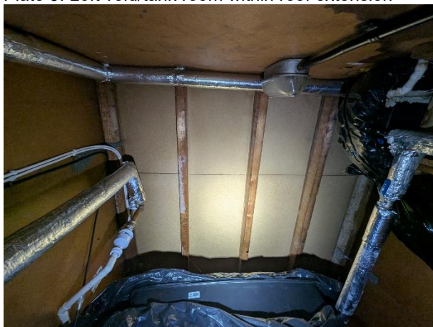
Plate 9: Loft void/tank room within roof extension
