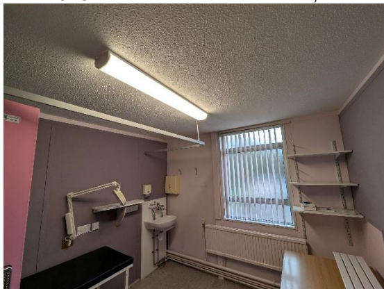
Plate 13: One of the examination rooms, all were very similar.
