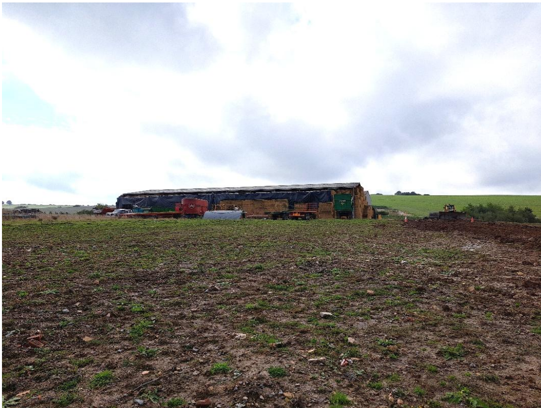
Photo looking south towards existing building (No.5) showing extent of land re-profiling
