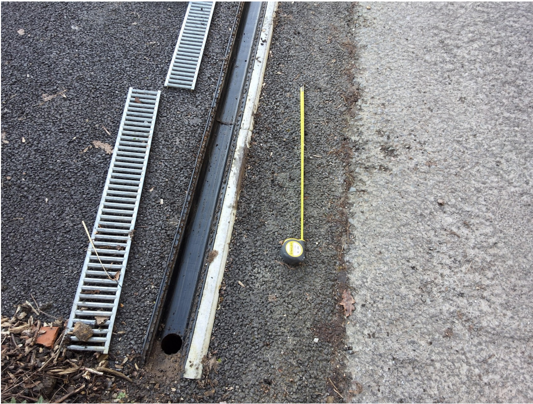
3. Emptied of debris and cleaned Aco drain at toe of drive demonstrating running outlet at lowest point
