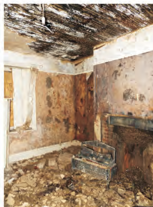
Typical condition of the interior of the house
