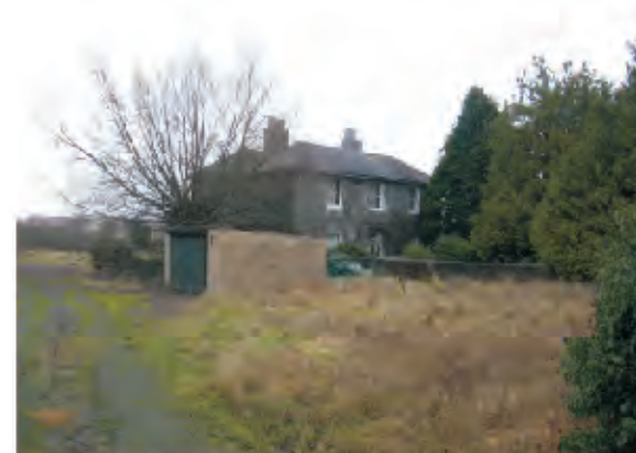
The house from the west, with garage in front.
