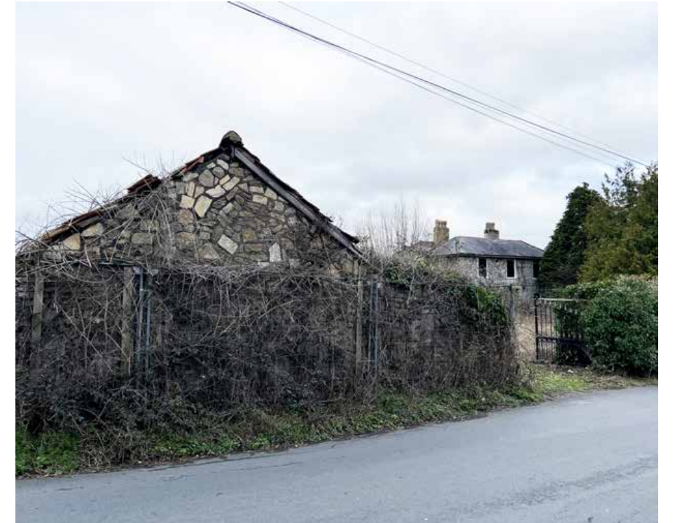
Photograph 6. View from Drynham Road, looking towards the Site, with the existing barn building in the foreground and farmhouse building in the background.
