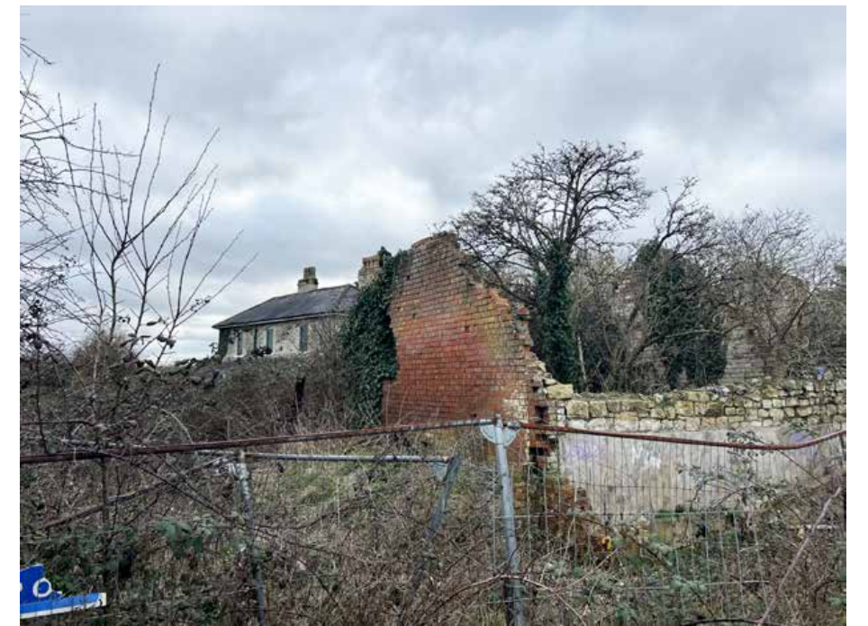
Photograph 15. View from the footpath looking towards the Site boundary with the barn building and fencing in the foreground, with overgrown vegetation and farmhouse building in the background.
