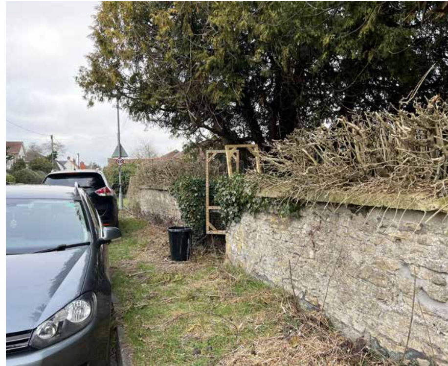
Photograph 5. View of the existing wall and opening of the farmhouse garden area from Drynham Road.
