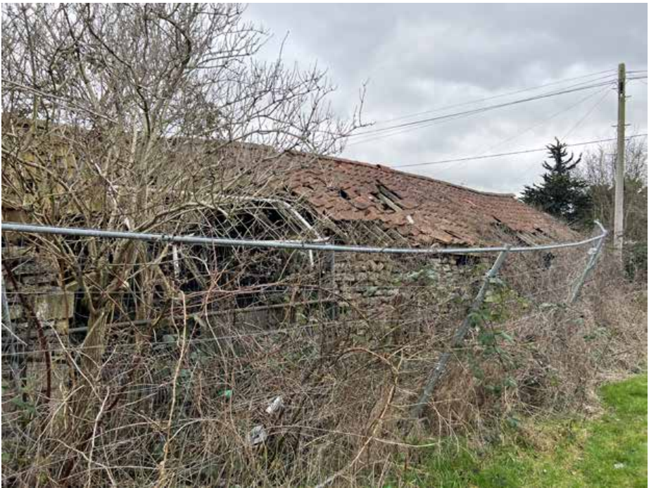
Photograph 4. View from the footpath, looking towards the existing barn building and Site boundary.
