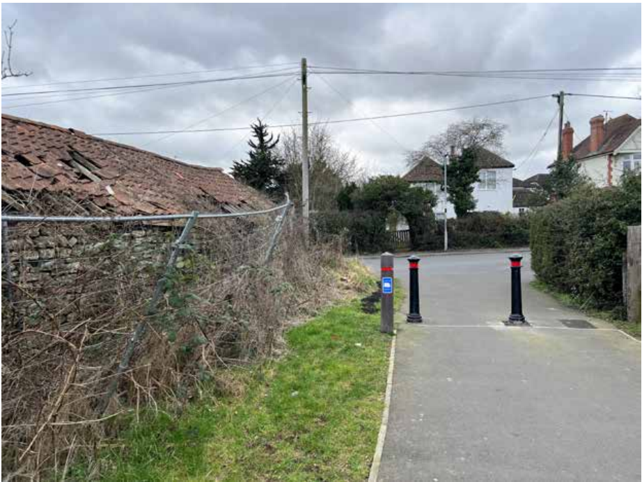
Photograph 3. View from the footpath, looking towards the footpath entrance, existing barn building to the Site and residential properties along Drynham Road.
