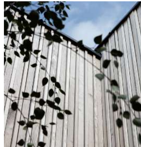
Articulated Cladding - Allowed to weather and silver.
