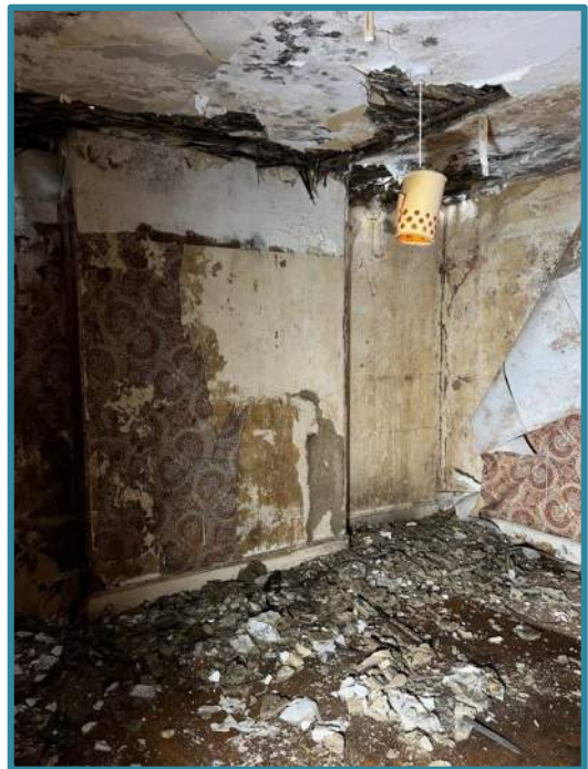
Figure 23 – Daylight visible through central valley soffit
