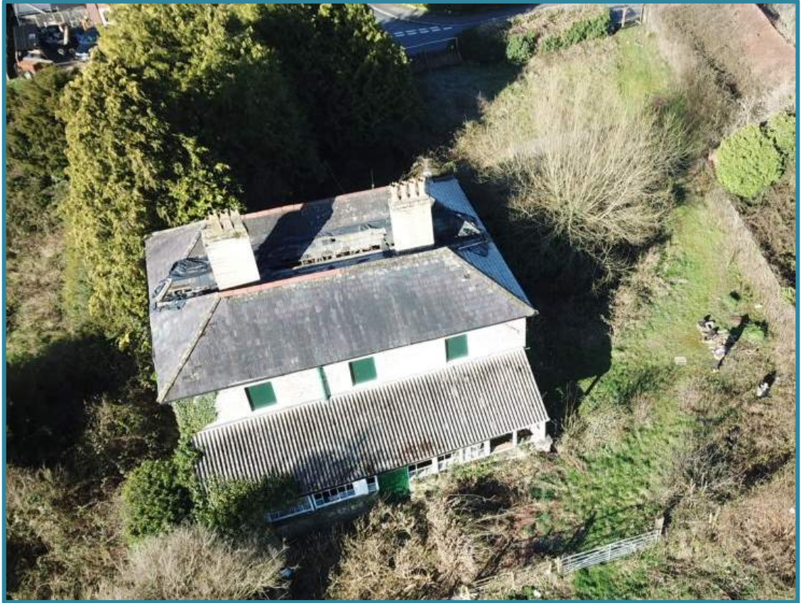
Figure 1 Farmhouse – aerial view from northeast aspect
