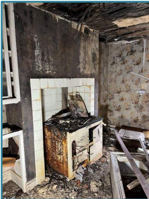
Figure 10 – G.F. Room 1 (North) Kitchen
