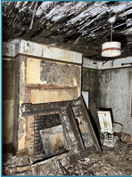
Figure 16 – G.F. Room 4 (South)
