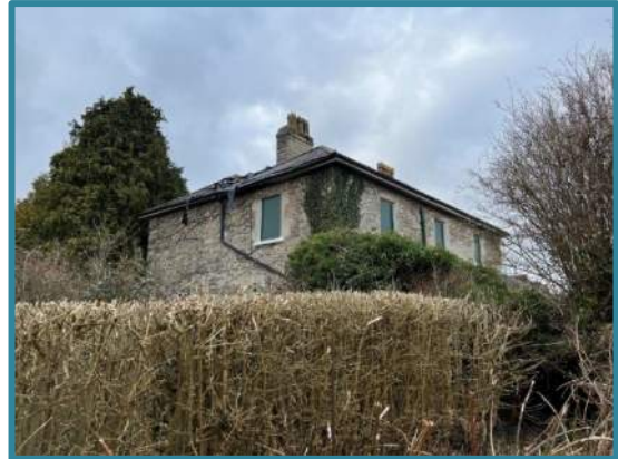
Figure 5 – View from east side
