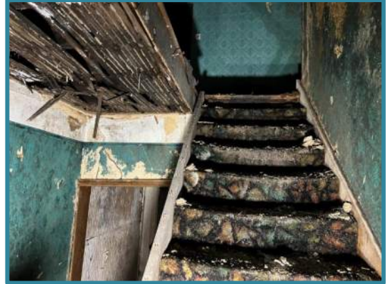
Figure 17 – Stair to First Floor
