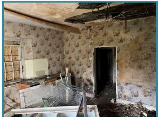
Figure 11 – G.F. Room 1 (North)
