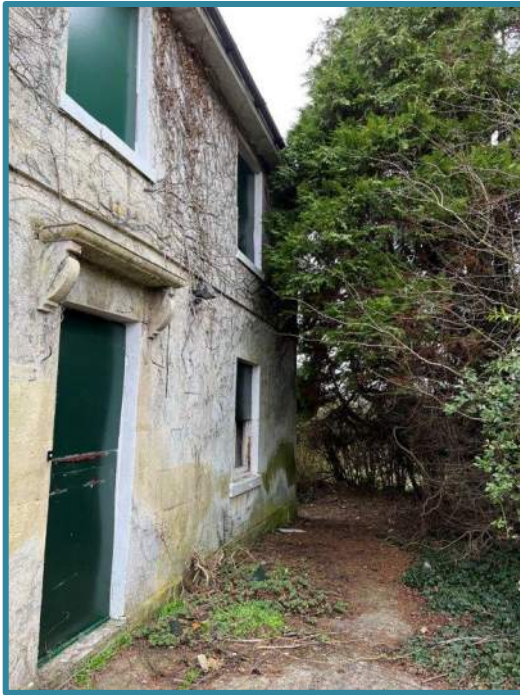
Figure 28 – Front ashlar façade (southwest)
