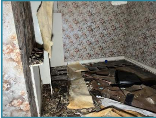
Figure 20 – F.F. Bedroom 1(North)
