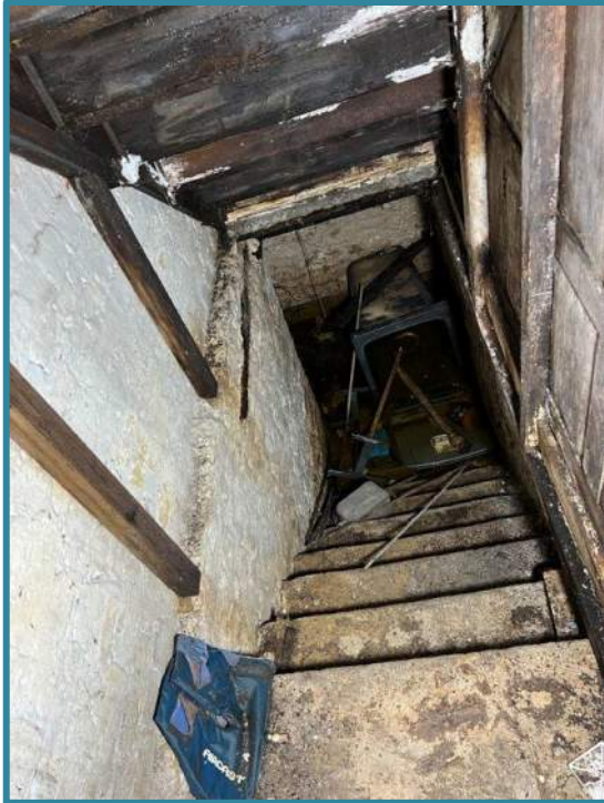
Figure 8 – Steps to (partial) basement
