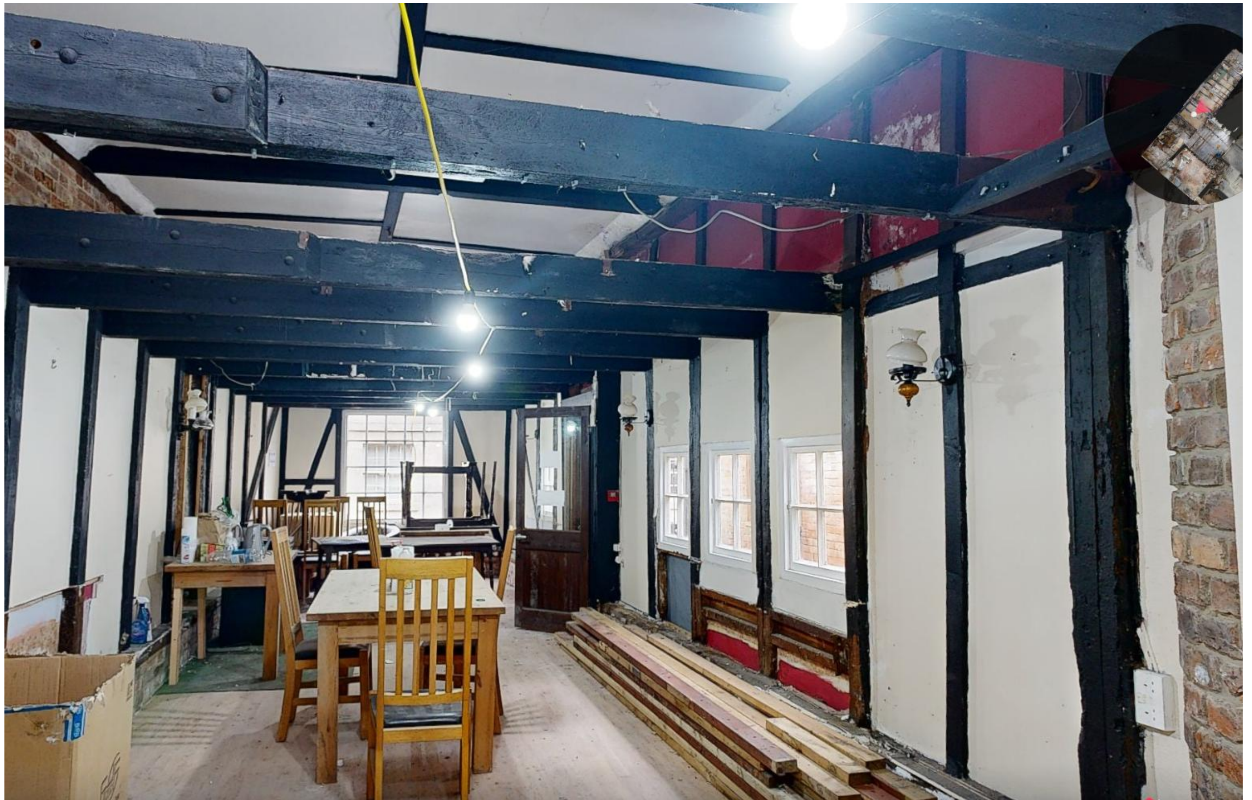
Photograph showing interior of outbuilding. Note some historic timber to internal face of courtyard elevation although originality unknown. Image taken from Matterport scan.
