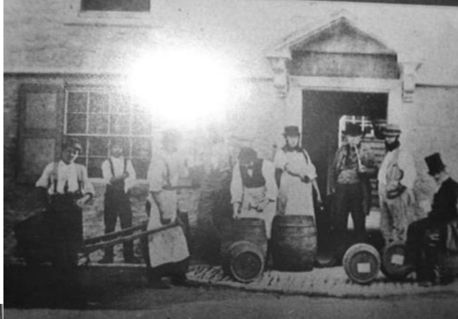
Copy of photograph of The Carpenters Arms held by the Wiltshire Building Records – file No. B3029.
