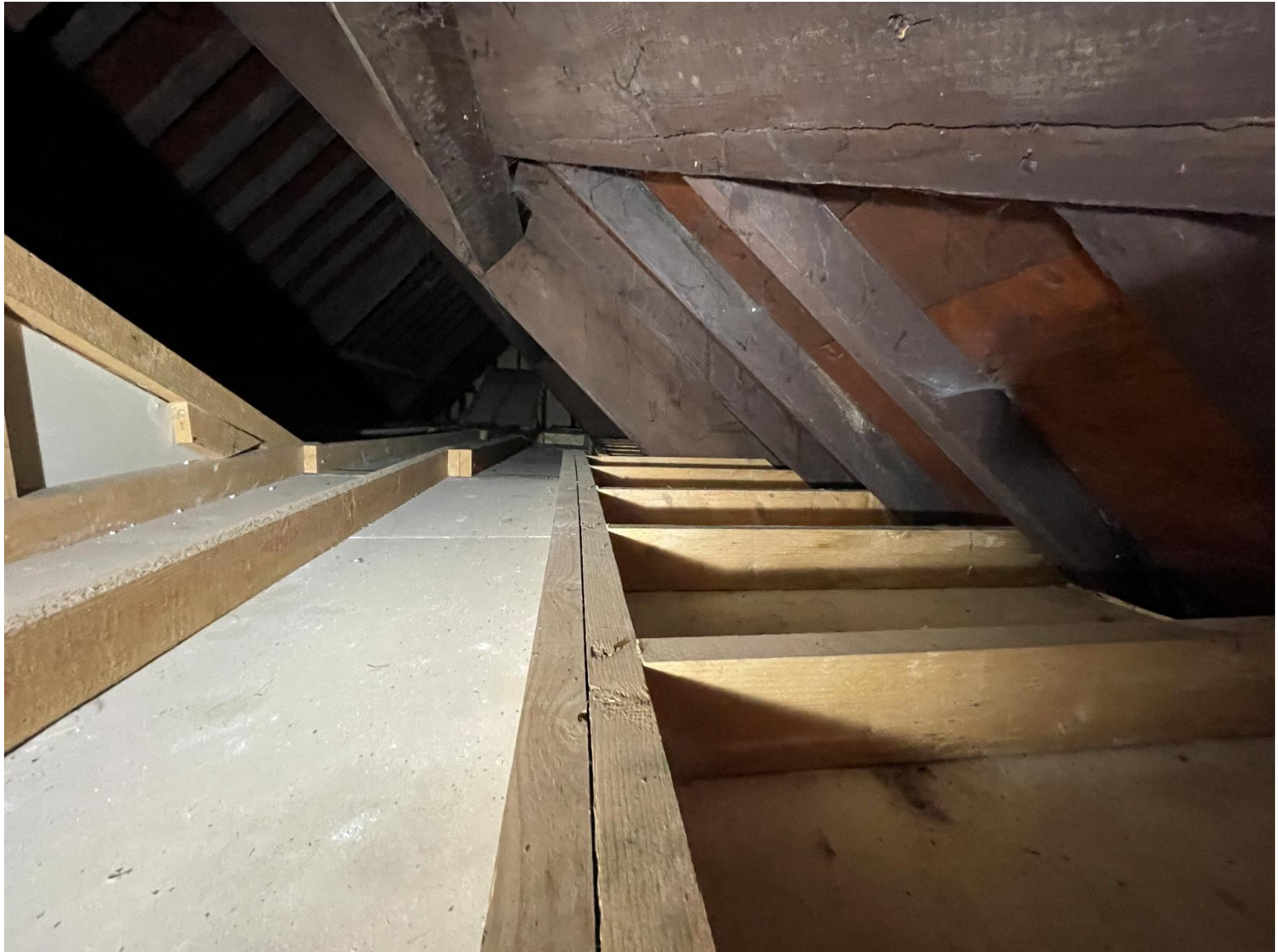
Photograph showing roof structure of outbuilding. Modern sawn timber throughout.
