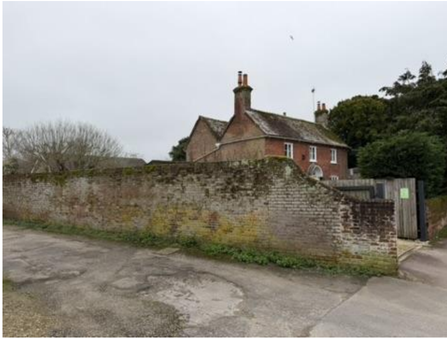
Photo 3. View from the Headlands and A338. The proposed building will fill that portion of sky between the tree to the left and the house, almost to the height of Radnor House.
