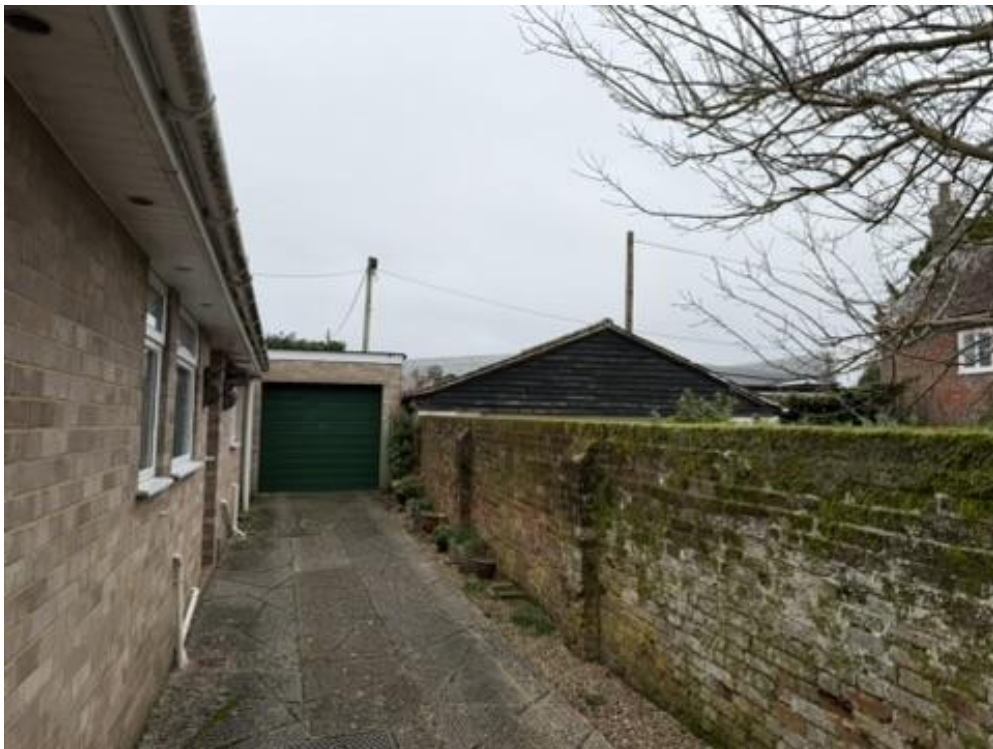
Photo 2. The front entrance and driveway to No 6 The Borough showing the proximity and position of the current outbuilding.
