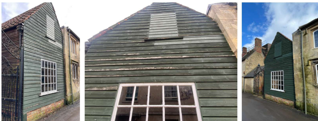
Existing timber structure proposed to be replaced
