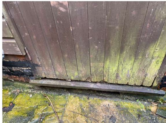
Stepped threshold to existing outbuilding
