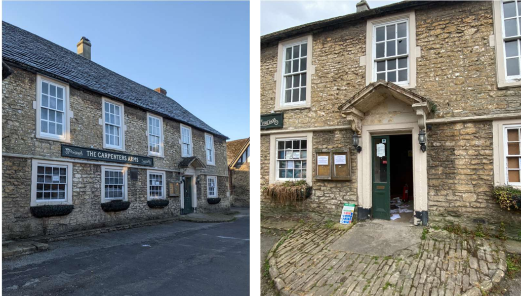
Photos of the existing flag stone strip and curved apron to main entrance
