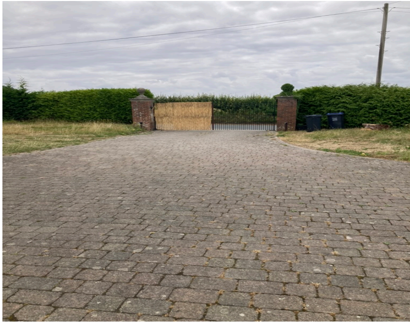
Existing wide vehicular access with brick piers and gates at Wheatlands
