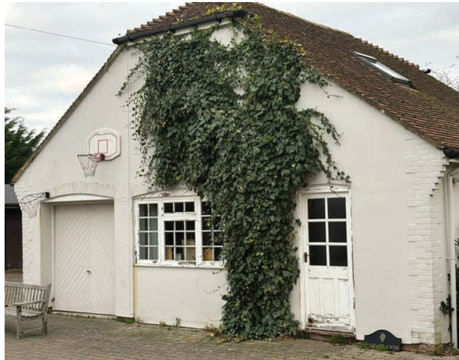
Fig.3 Photo of west elevation two storey residential annex/garage
