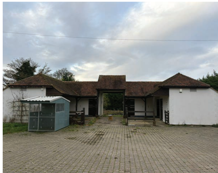
Fig.6 Photo of south elevation of stables
