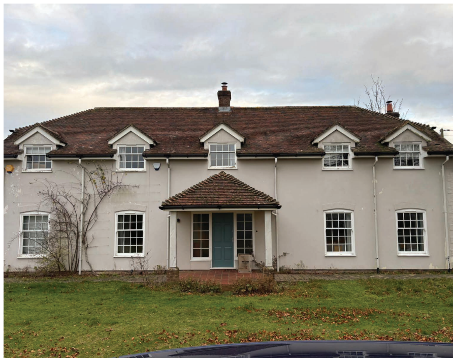
Fig.5 Photo of west elevation of main house
