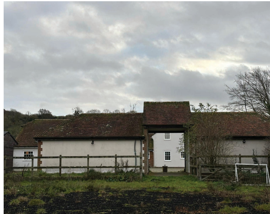
Fig.4 Photo of north elevation of stables
