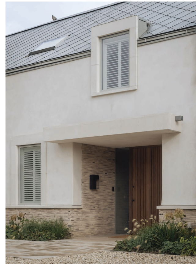
Fig.20 New build house completed in Houghton, Hampshire, 2024. Winner of British Home House of the Year 2025
