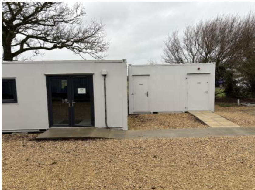
Toilet building marked 9 on the aerials image inserted previously
