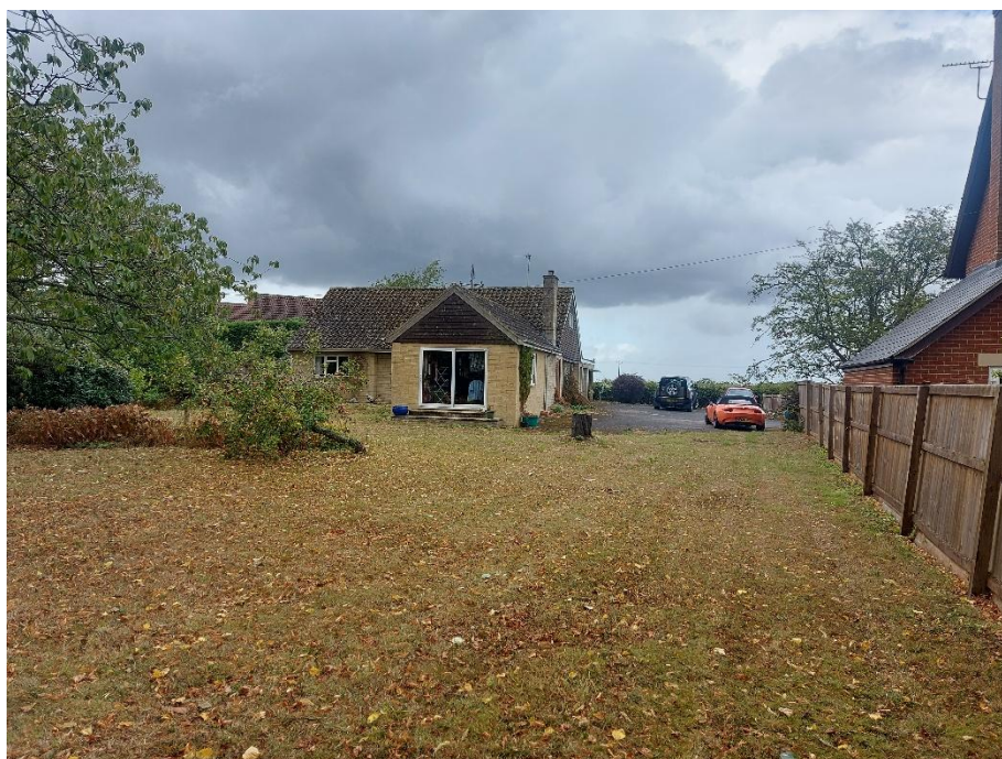
Figure 4: Photograph of Three Ways and its parking area – view looking north
