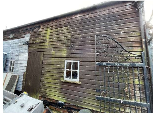
2.12) Modern fixed casement windows and a modern close boarded stable door.
