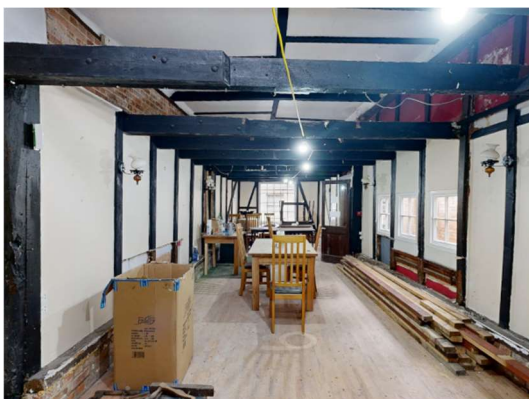
3.1) Interior view looking West towards East St. Plasterboard ceiling above the intermediate joists with applied faux timber detailing.
