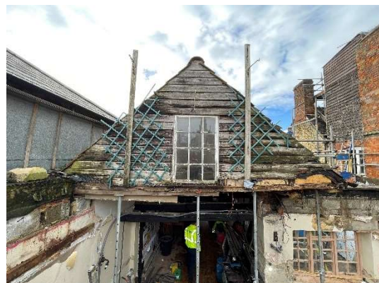
2.4) East facing gable, the gable was supported on the flat roof structure that has been removed in the photo and is to be replaced.
