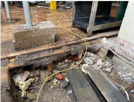
3.11) The floor is a modern engineered timber board on tongue and groove floor boards that are laid over a fibrous material over chipboard on joists. There is no evidence of a cement floor at the western end of the building (as should have been installed as part of the previous permission works).
