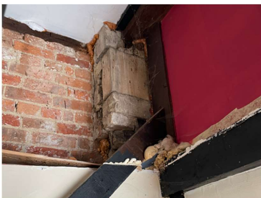
3.7) Abutment to neighbouring stone building. Modern block and foam seen.
