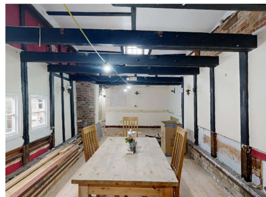
3.2) Interior view looking East.
