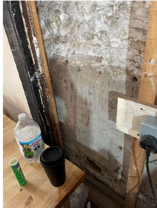
3.10) Painted stone wall with cementitious render at low level behind plasterboard lining. Extent of cementitious render unknown at present.
