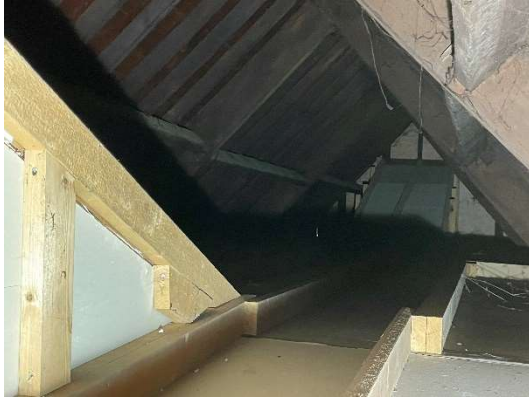
4.1) The roof is formed of simple trusses with purlins spanning between, supporting rafters. Access to the roof void is limited and further investigation is needed to ascertain the age of the roof timbers. Rafters are over-boarded with timber sarking board.
