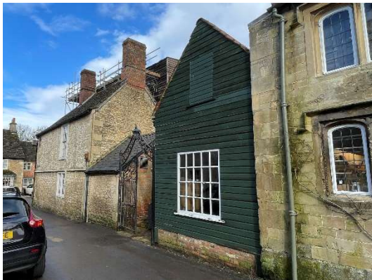
2.1) East St. Elevation with timber clad gable. The lower window is a modern casement. The high level window has been boarded over, and a modern casement remains behind the cladding boards.
