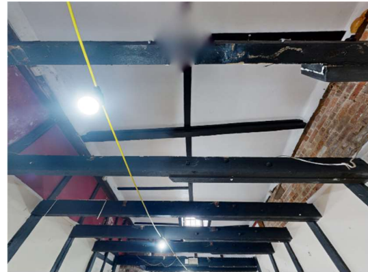
3.6) Plasterboard ceiling with truss chord visible and applied timber decorative detail.
