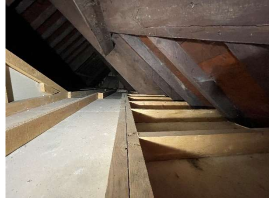
4.2) The ceiling is modern plasterboard on softwood framing between the trusses. At each end there is a hood formed in plasterboard around the high-level windows.
