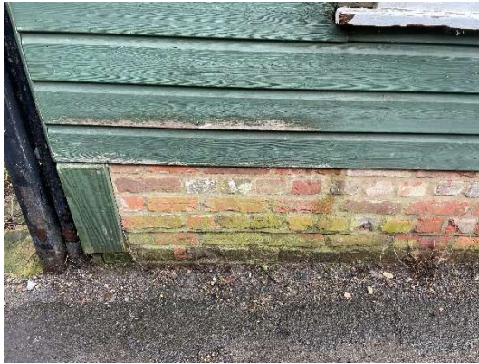
2.9) The gable facing East Street has a brick plinth in modern brickwork with cement mortar and a dpc.
