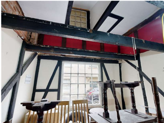
3.5) Fixed casement window to gable and high level window overboarded externally.
