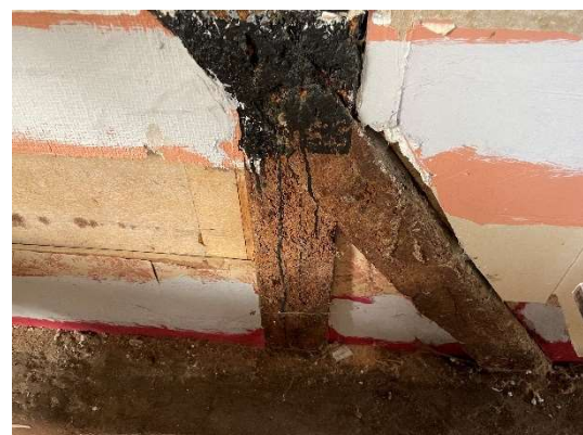
3.8) Where radiators have been removed, some historic timber framing is visible with modern materials used for infill panels.
