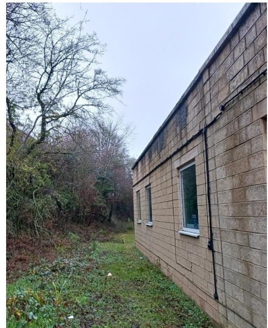
Photo 12 Existing structure off-site
