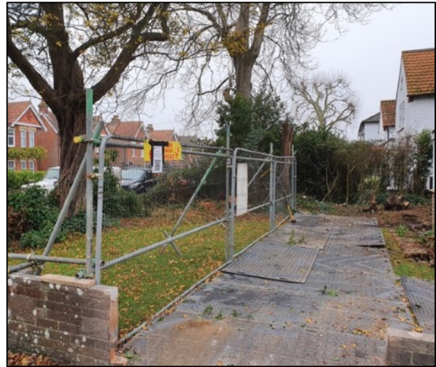
GP2: Tree protection barriers & trackmat ground protection
