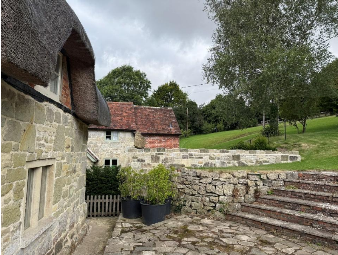
Fig.6 Rear of The Rookery looking across to Deer Cottage – steps behind wall.
