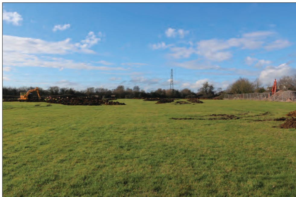
Site looking west
