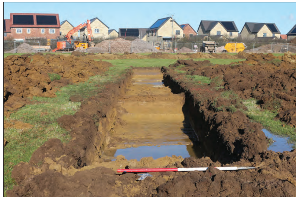
Trench 10, looking north-east (1m scale)
