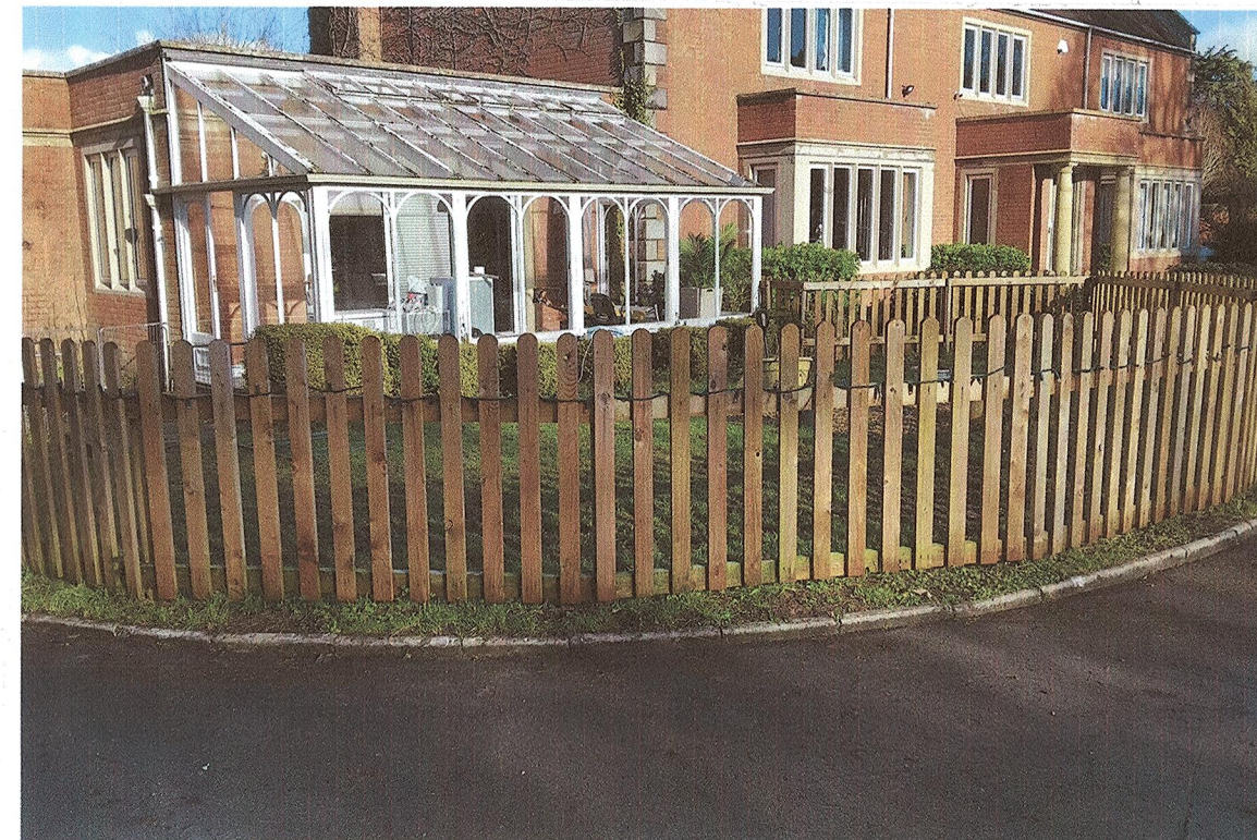
GENERAL PICTS - SHOWING CONSERVATORY - WHICH IS TO BE DEMOLISHED & EXIST. 'WICKET-FENCED' EDGING AROUND DRIVEWAY.
