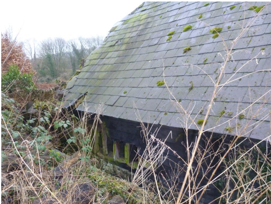
Fig 4: Barn A is open to the elements on most faces.
