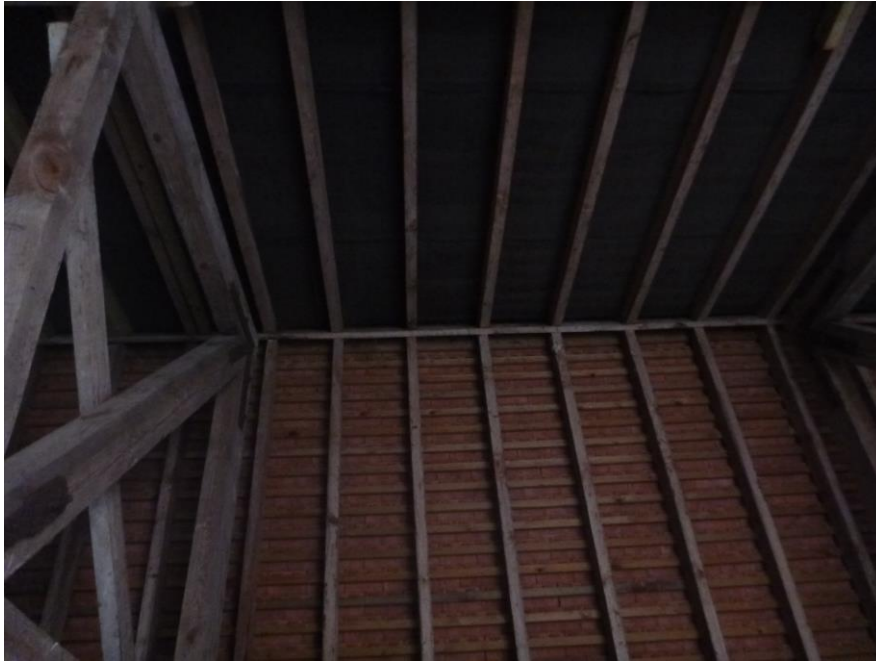
Fig 9: The southern pitch of the roof is lined with bitumen felt and the northern face is unlined.
