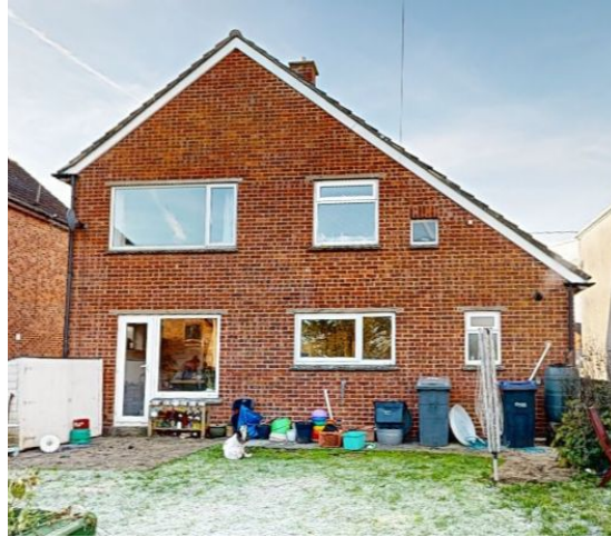
Existing Rear facade
