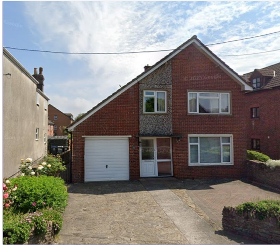
Existing Front facade
