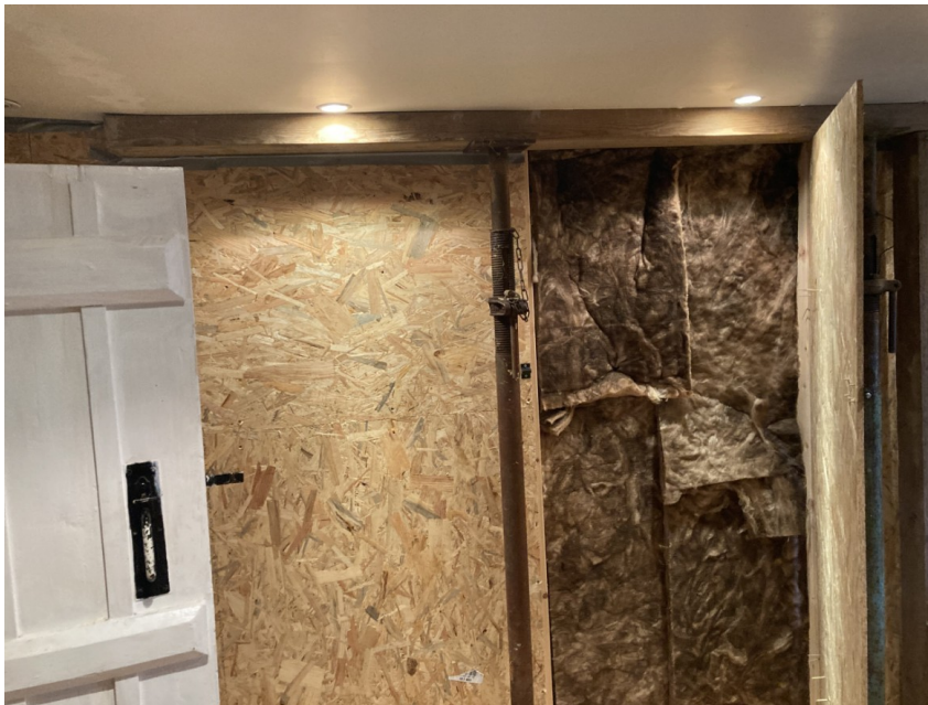
2. Temporary propping installed internally.
