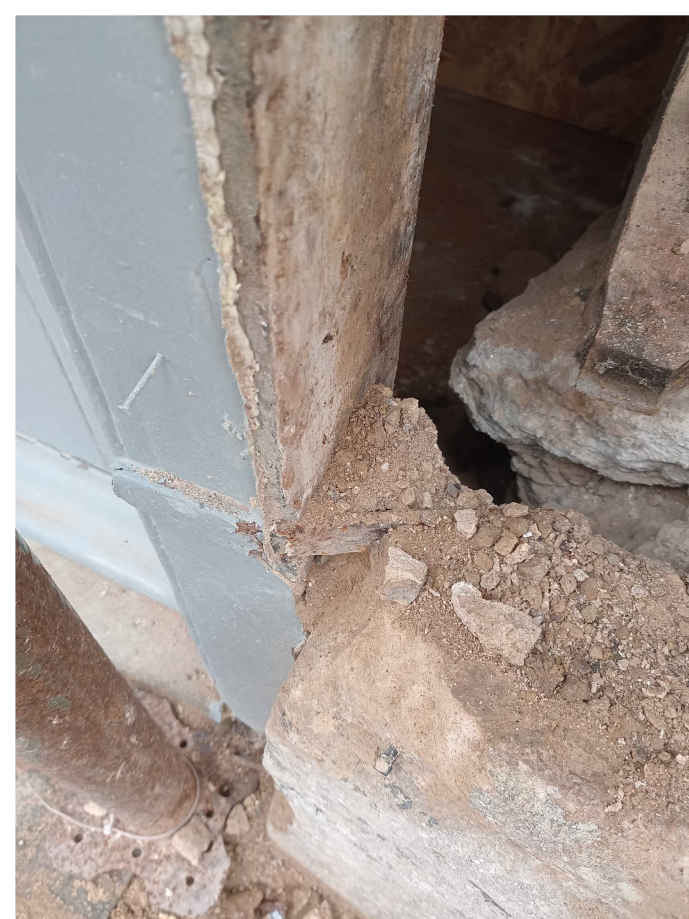
Photo 3: Photo of metal straps to door, keyed into the wall
