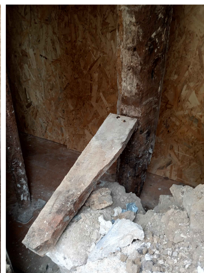
Photo 5: Photo showing timber wall ties
