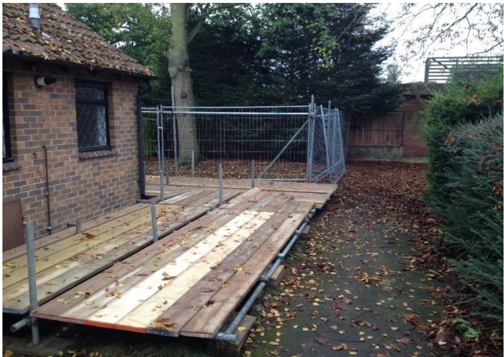
Figure 7 – Specification for scaffold ground protection
