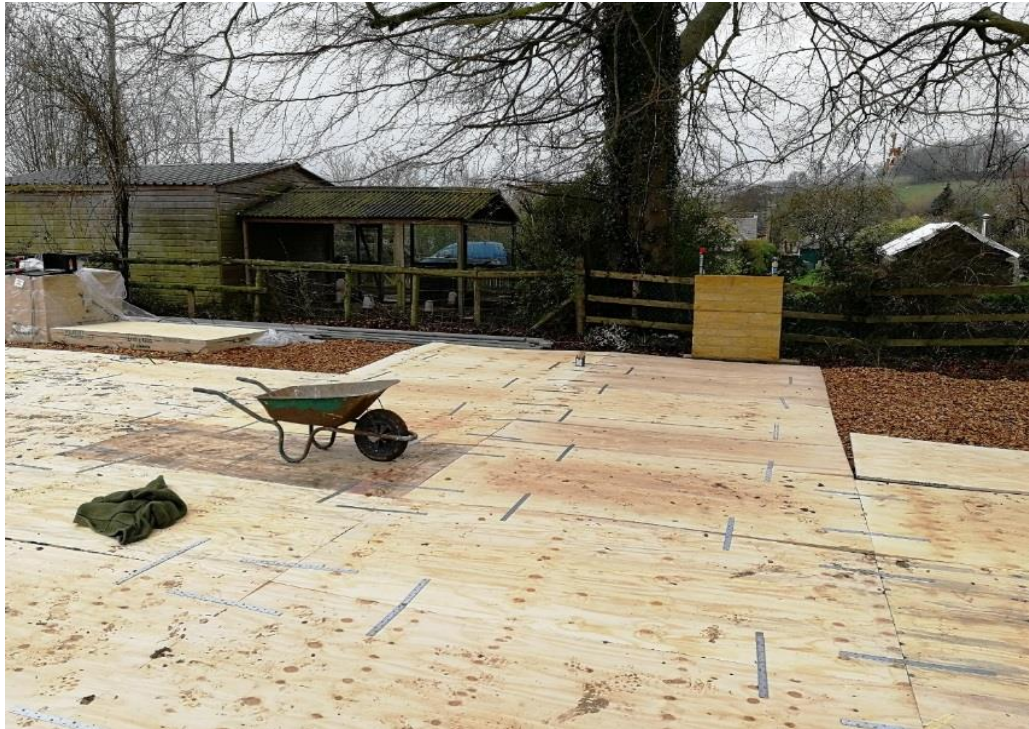
Figure 6 – Plywood sheeting used as ground protection.
