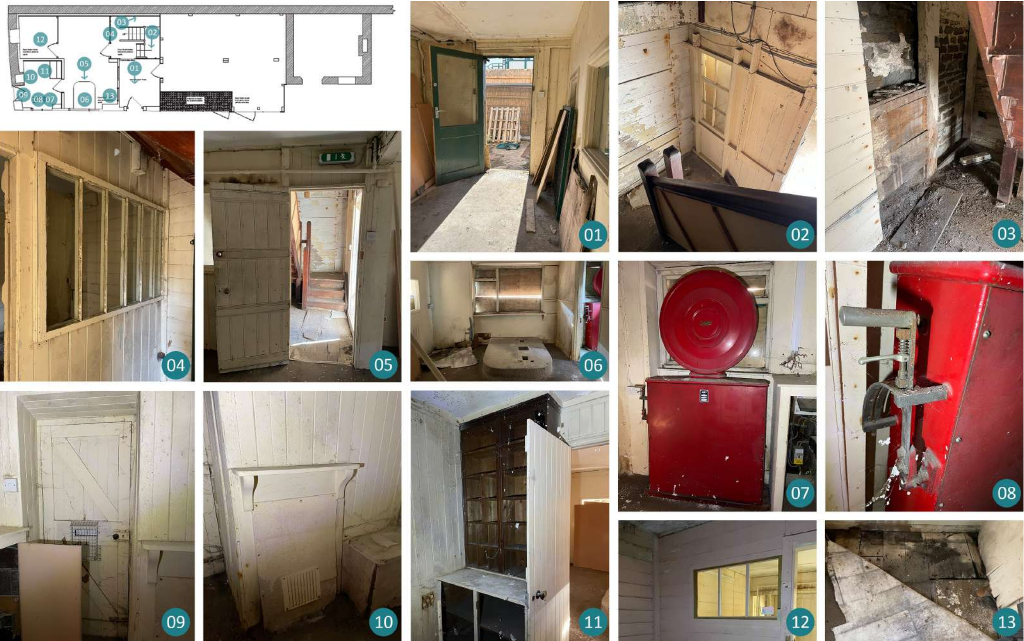
FIG 09: Internal images rooms 02-06 (ground floor)
