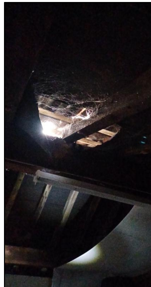
Photo 8 Hole in loft void felt
