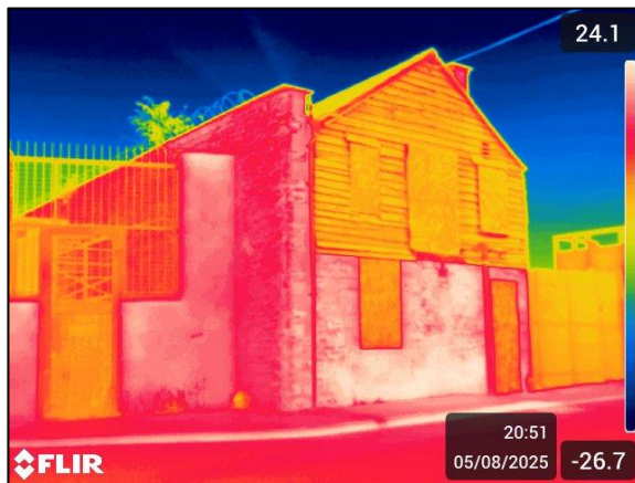
Photo 11 North west elevation
