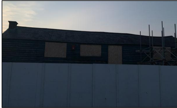
Photo 1 Southern elevation with security fence
