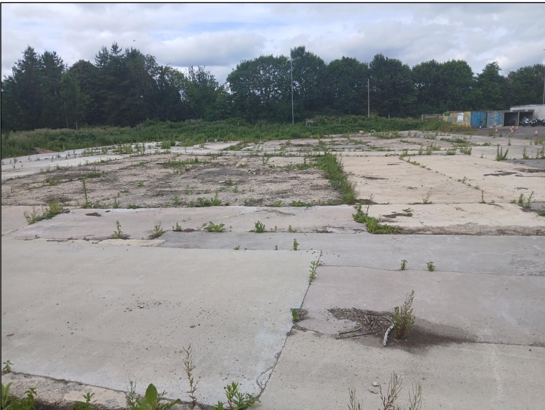
Photograph 6: View facing northwest showing underlying concrete beneath tarmac and southwestern boundary.
