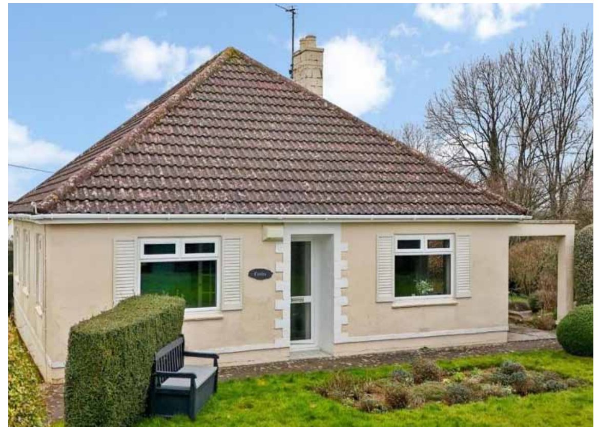
Close-Up view of south elevation
