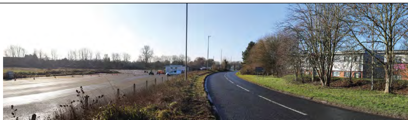
Figure 4-3: Views from London Road alongside the site (extract of Photoviewpoint 8a)
