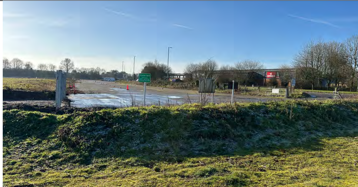
Boundaries and asphalt strip alongside London Road to the northeast of the site
