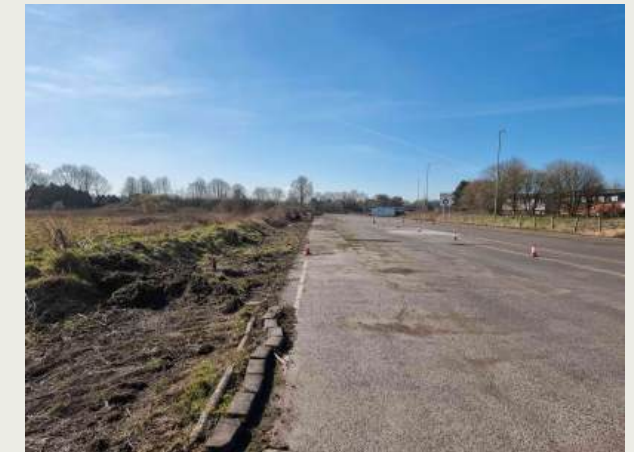
Image 2 – View of eastern boundary (Site photo March 2025)
