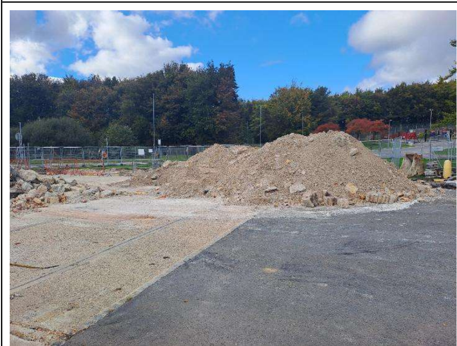
Photo 4: Stockpile of removed concrete and Made Ground in tank farm (8 th October 2025)
