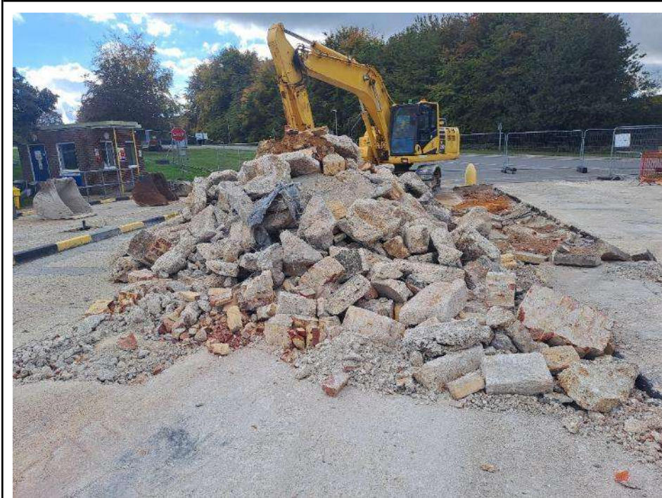
Photo 4: Stockpile of removed concrete and Made Ground in tank farm (8 th October 2025)
