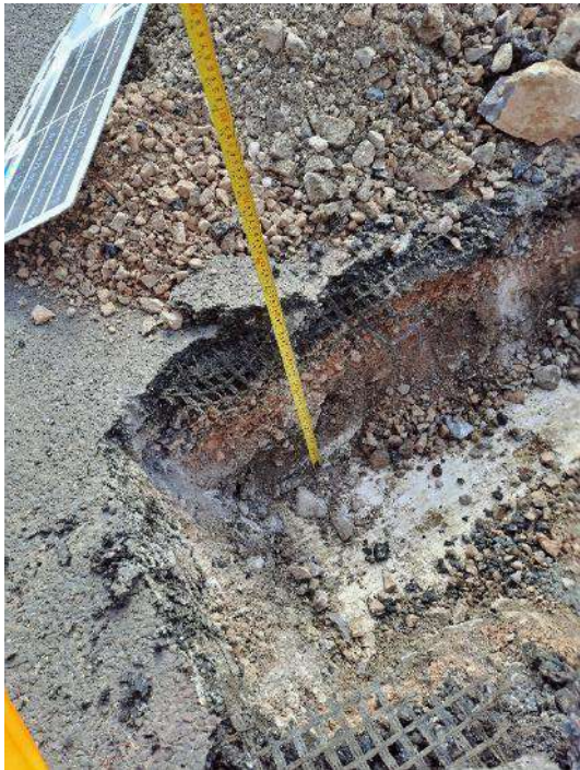
Photo 14: TP05 excavation. (5 th September 2025)
