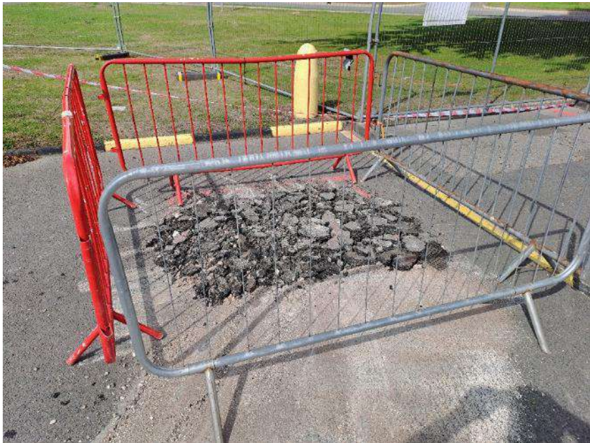
Photo 15: TP05 backfill (5 th September 2025)
