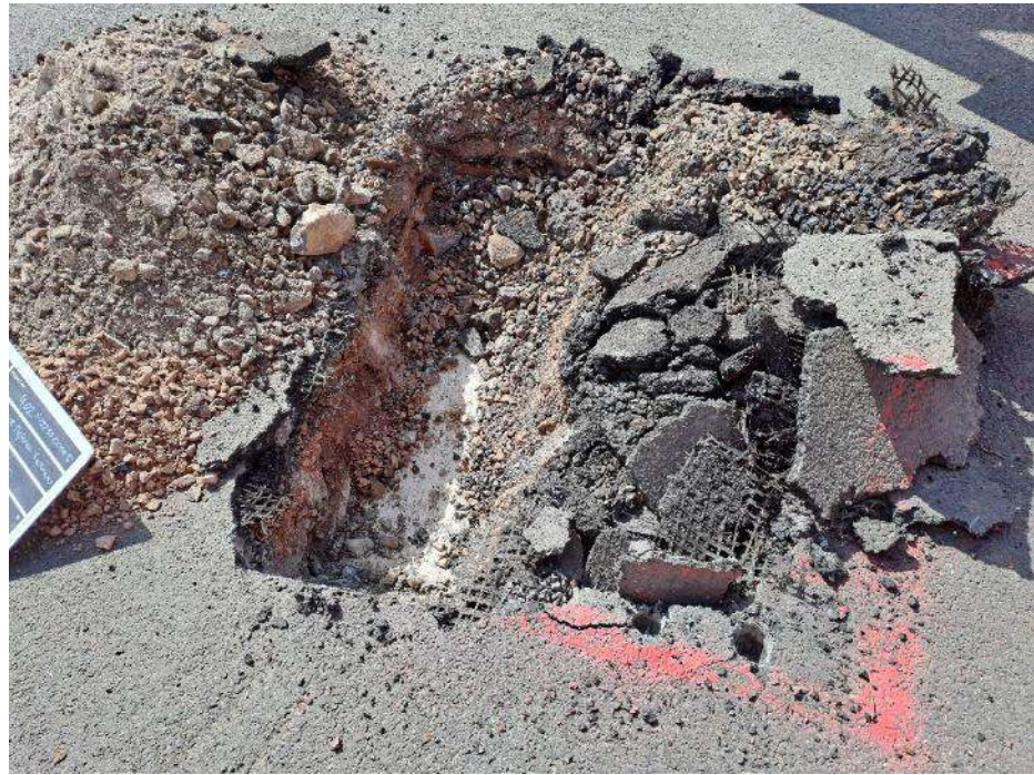
Photo 13: TP05 excavation and arisings. (5 th September 2025)
