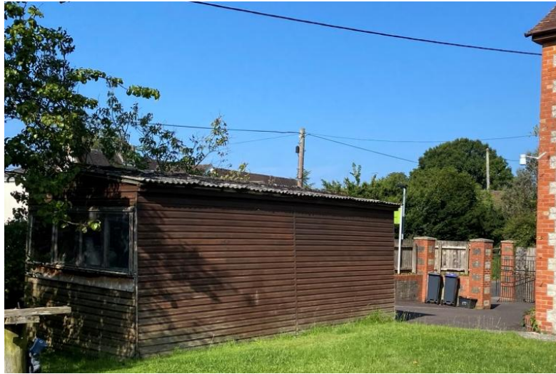
Fig.6 Timber shed at front of site to be removed
