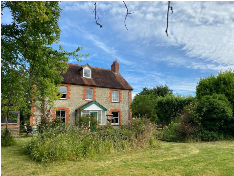
Figure 2: Southern elevation of Elmsleigh
