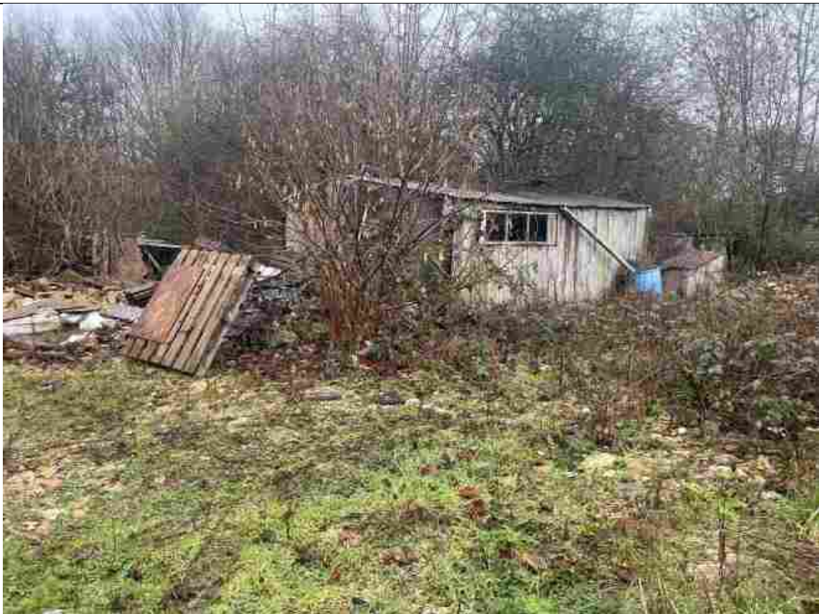
PLATE 2 – Dilapidated shed on western side of site by the access track with old building materials.
