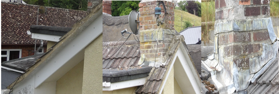
Figure 9/10. Composite covered roofs.
