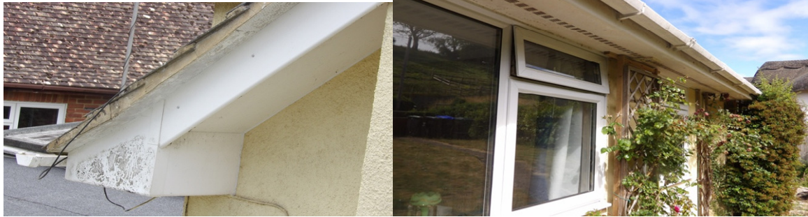
Figure 6. Example of eaves tiles. Figure 7/8. Leadwork around chimney.
