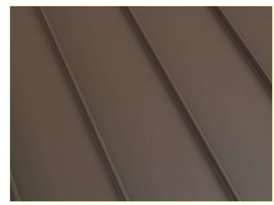
BROWN METAL STANDING SEAM ROOF
