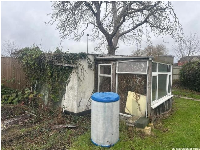
Photo 4: Garage (B2) present in the west of the site.
