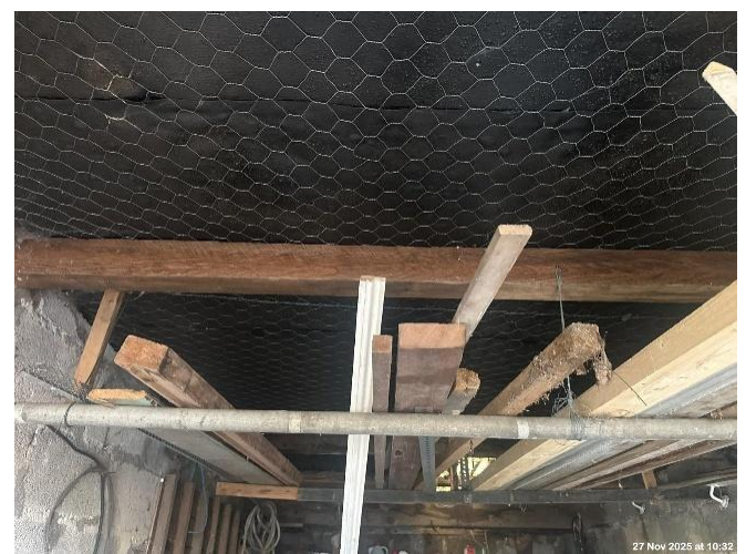
Photo 6: Inside garage (B2).
