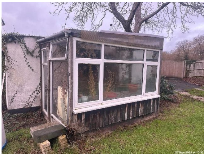
Photo 7: Conservatory on garage (B2).
