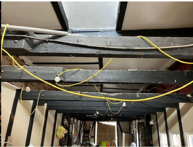
Figure 5 showing bolted cross beams
