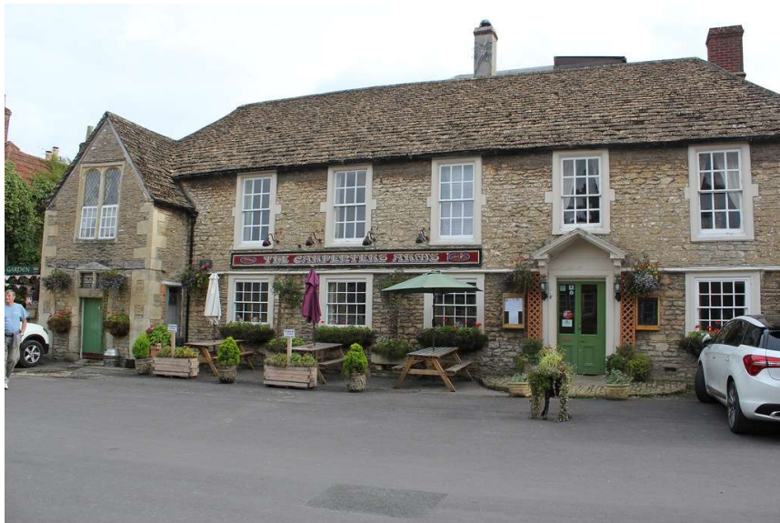
Figure 1: The Carpenters Arms, Church Street façade – date unknown.
