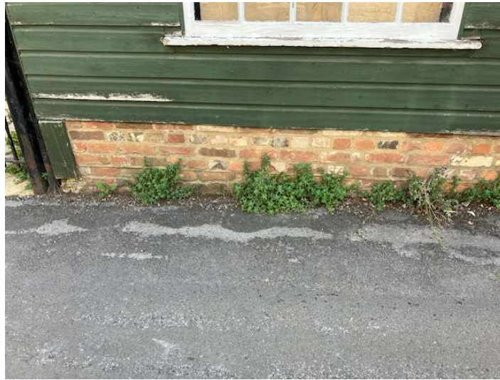
Figure 6 Modern DPC and recent brickwork.
