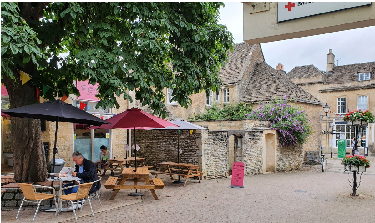
View from shopping precinct taken 2023 showing the opening in the southern boundary wall where the gate is to be installed
