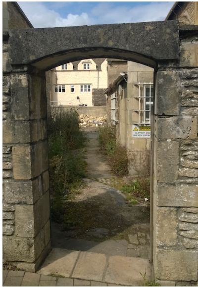
2023 photo of the opening in the wall.
