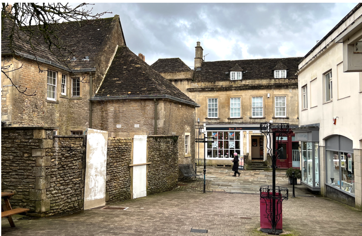
Current view with works active on site at 13 High St. Temporary protection is in place over the opening for site security until the gate is installed.
