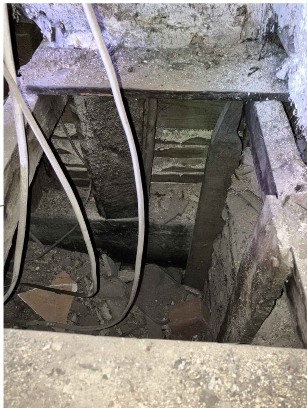
ORIGINAL TIMBER FRAME BEAM AND POST
