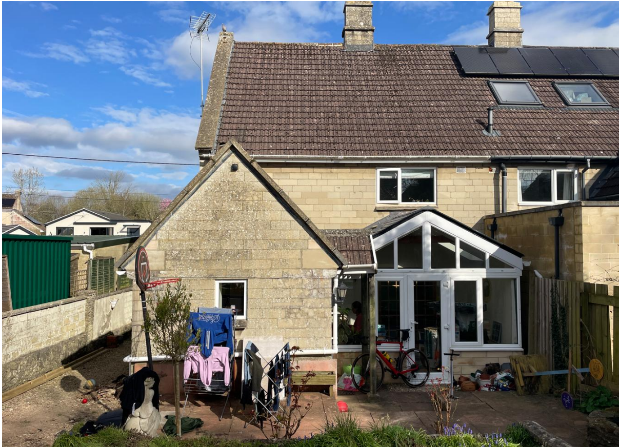
Current rear elevation to house
