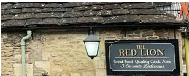
Guttering As Existing
