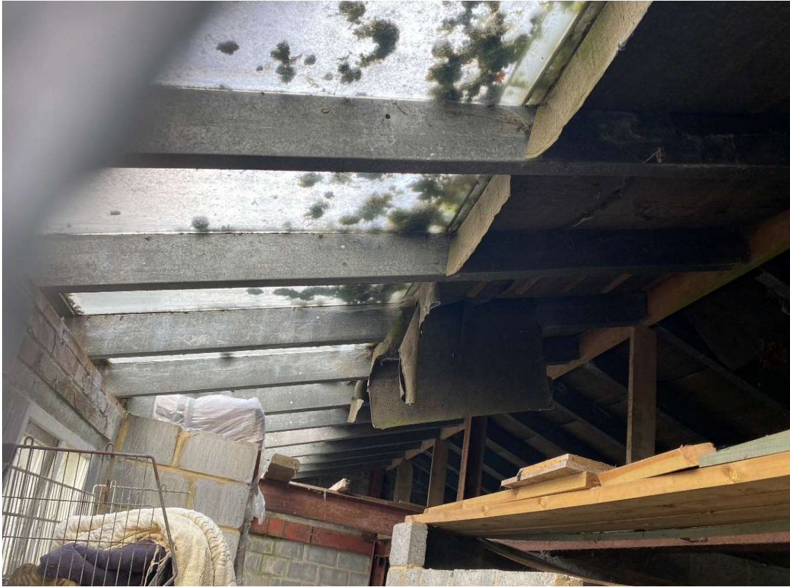
Figure 1.20– Underside of roof structure
