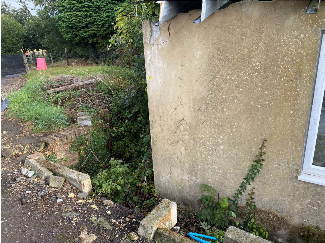
Figure 1.3 – Brick Retaining wall along gable
