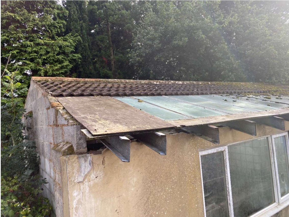
Figure 1.7– Roof slope with glazing and roof tiles
