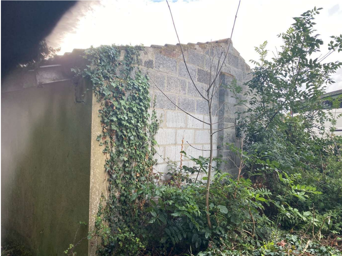
Figure 1.14 – Established vegetation along gable wall
