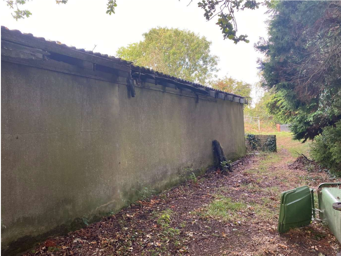
Figure 1.13 – Rear elevation – no gutters
