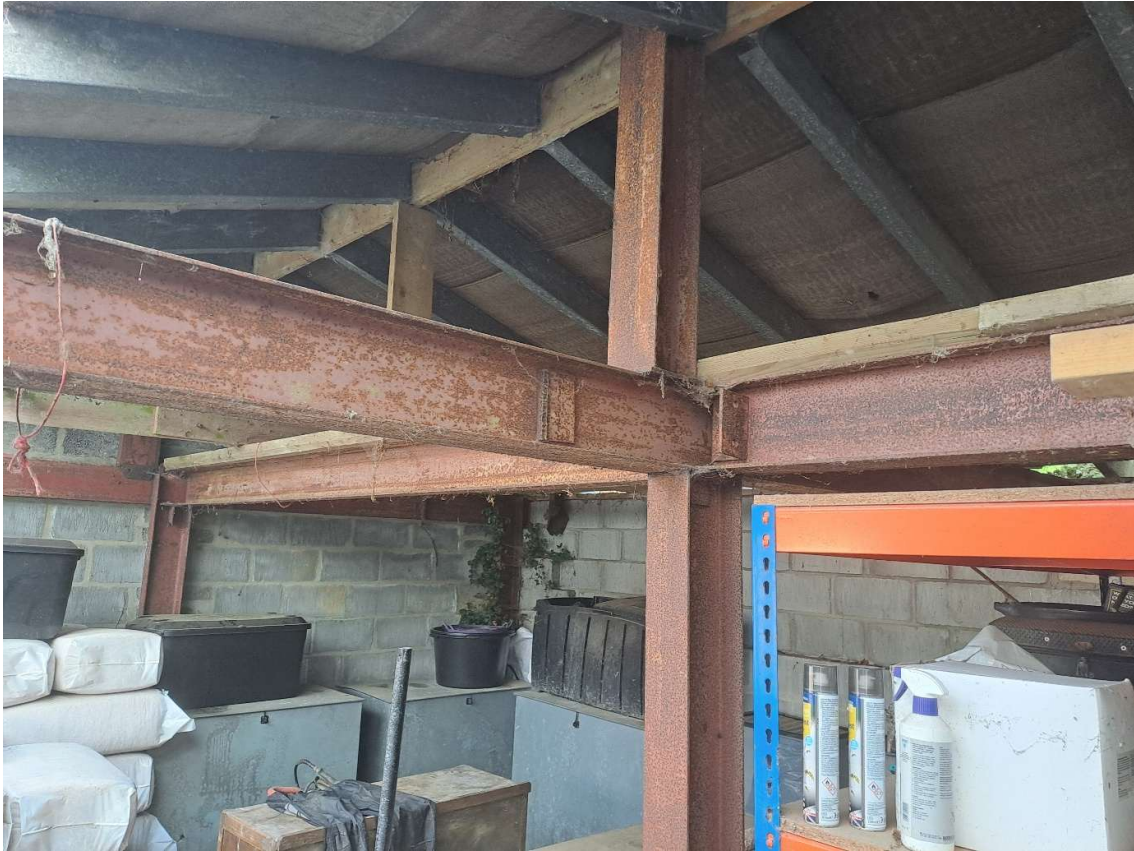
Figure 1.21 –Steel Framing supporting roof structure
