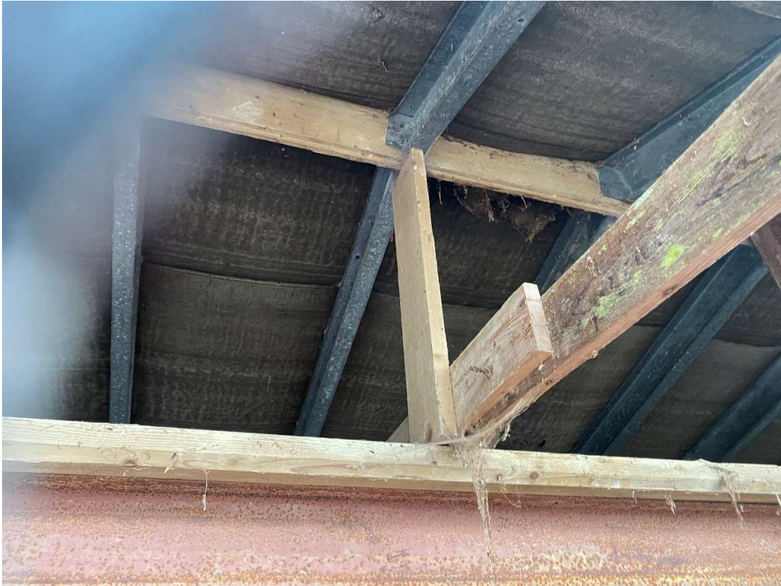
Figure 1.23 –Timber strut supporting roof structure
