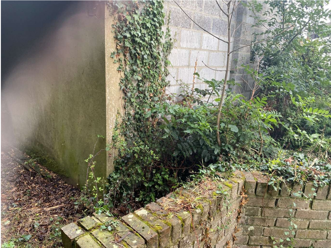
Figure 1.15– Brick retaining wall
