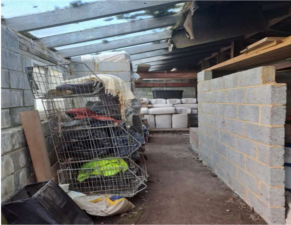
Figure 1.18 – Internal masonry walls
