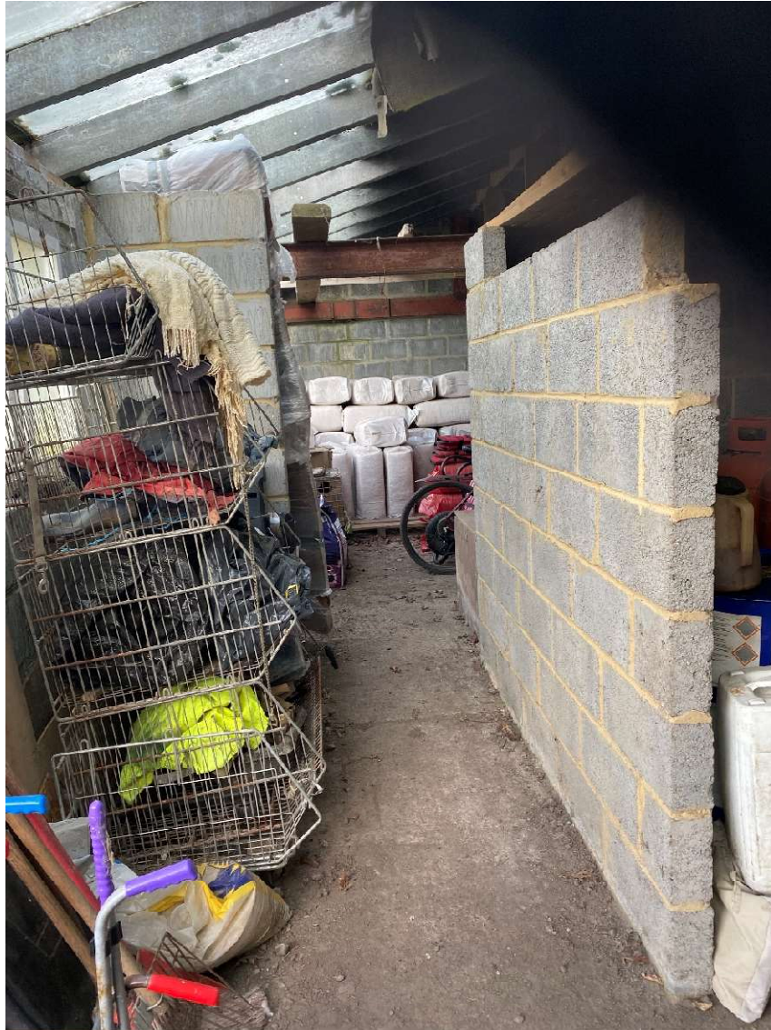
Figure 1.19 – Internal concrete floor
