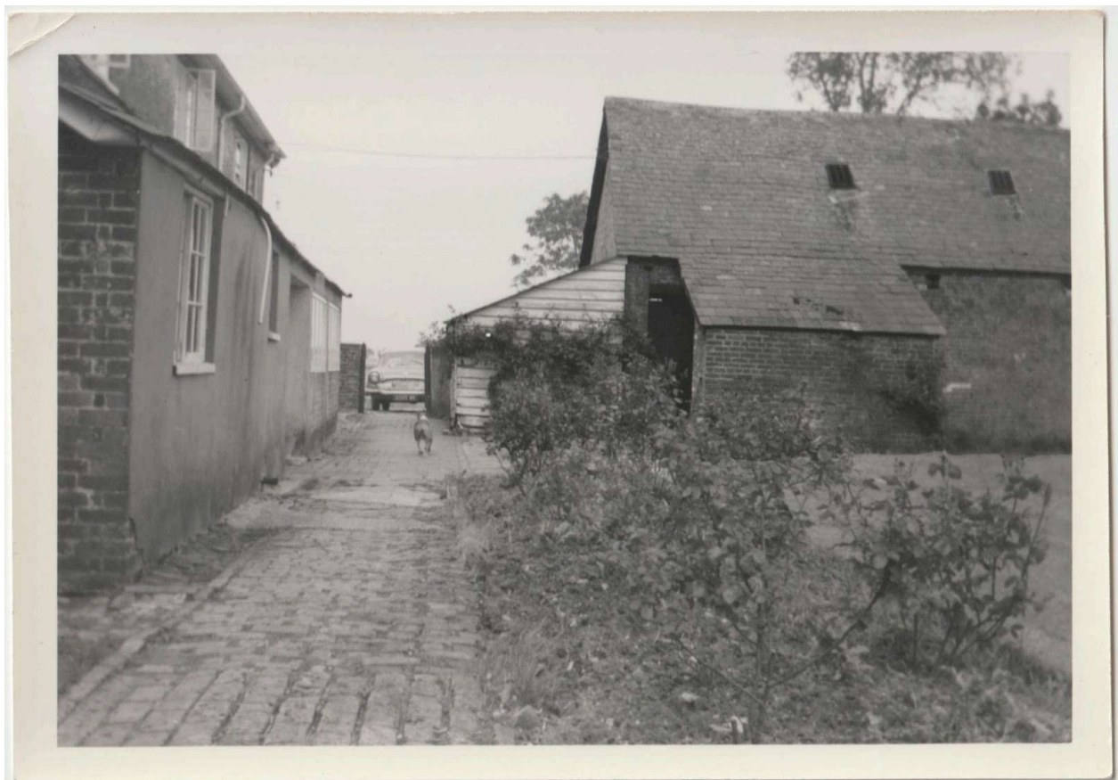
Fig 3. Rear view of The Coach house 1958. Previous roof lights visible on the rear roof slope.
