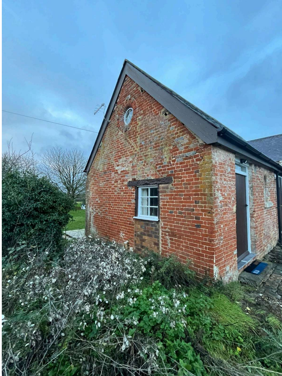
Fig 3. The Coach House southern elevation and retained original windows.
