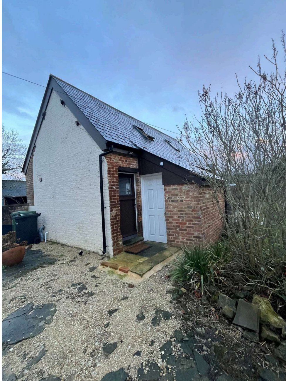
Fig 4. The Coach House northern elevation showing rear entrance door to the accommodation and door to separate boiler room.
