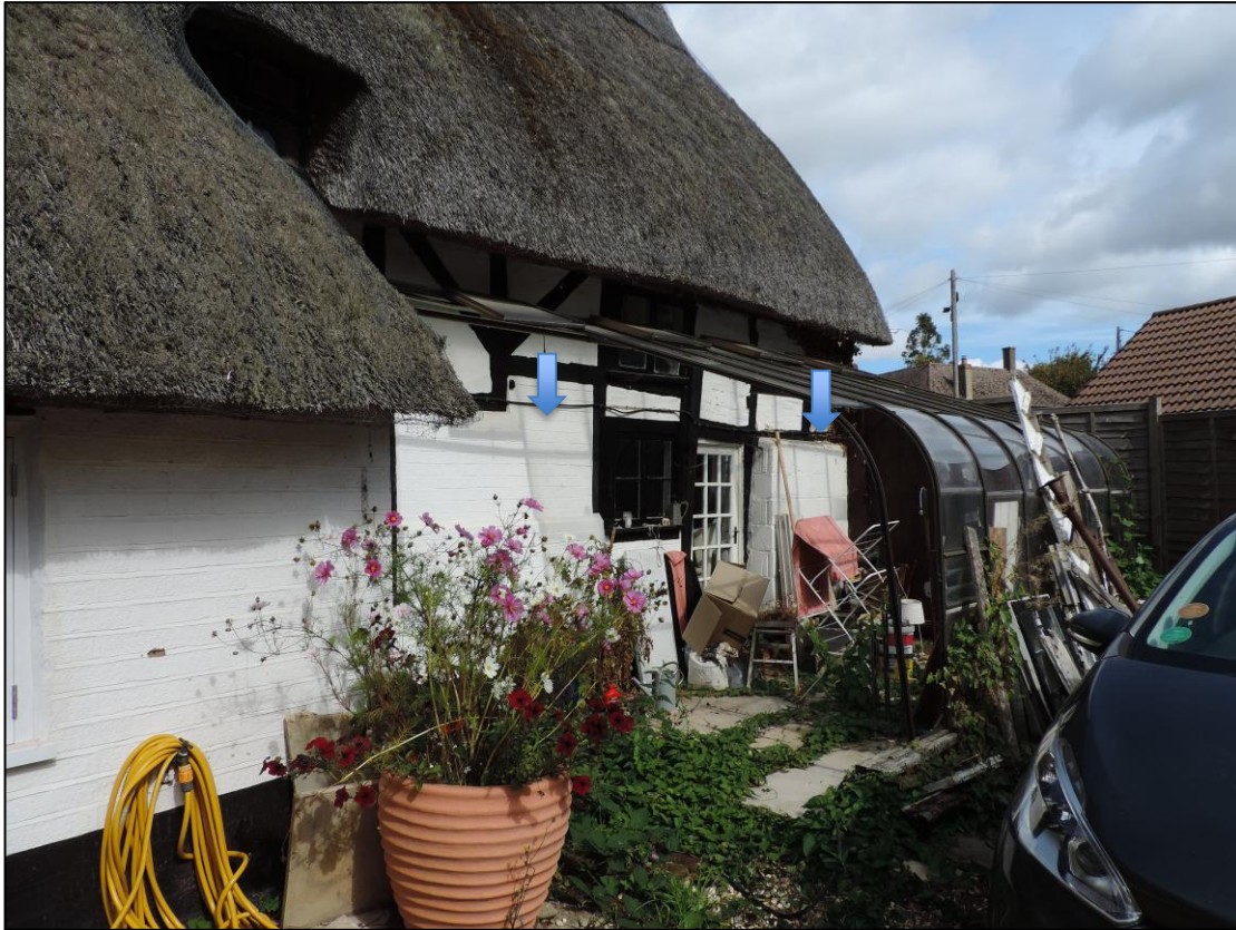
Photo 3 Northeast facing view of rear (south) elevation showing brick infill and cement block buttress.
