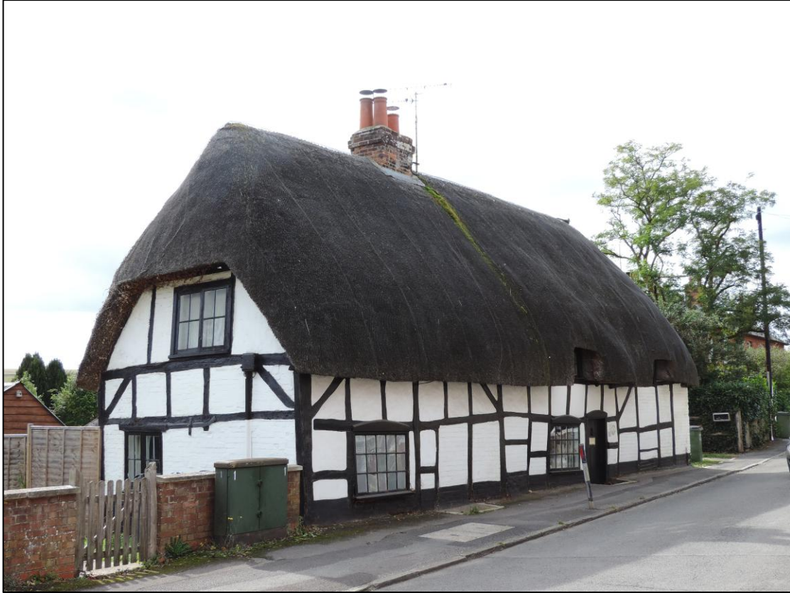
Photo 1 Southwest facing view of the principal (north) elevation of Jasmine Cottage from Oxford Street.
