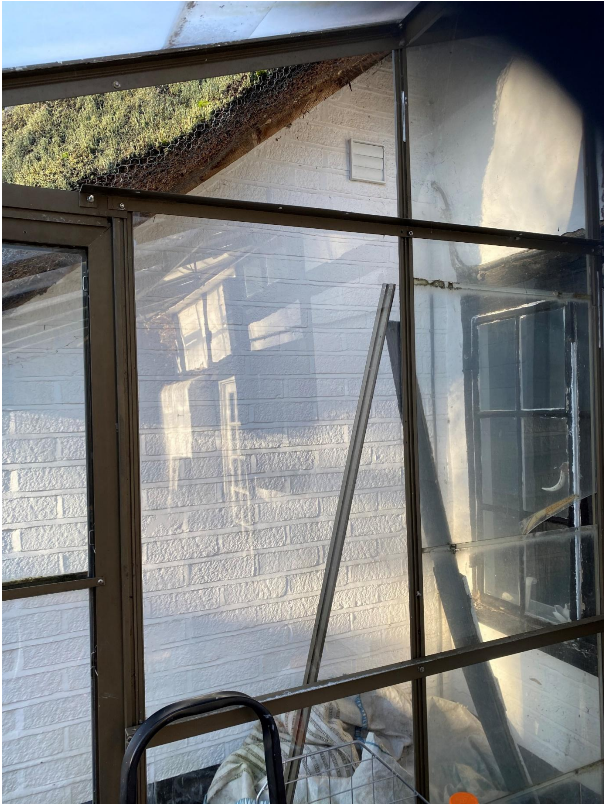
PHOTO 7 – REAR ELEVATION SHOWING THE INSIDE OF THE EXISTING CONSERVATORY
