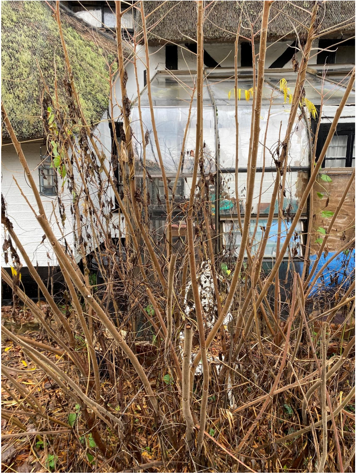
PHOTO 2 – REAR ELEVATION SHOWING EXISTING CONSERVATORY
