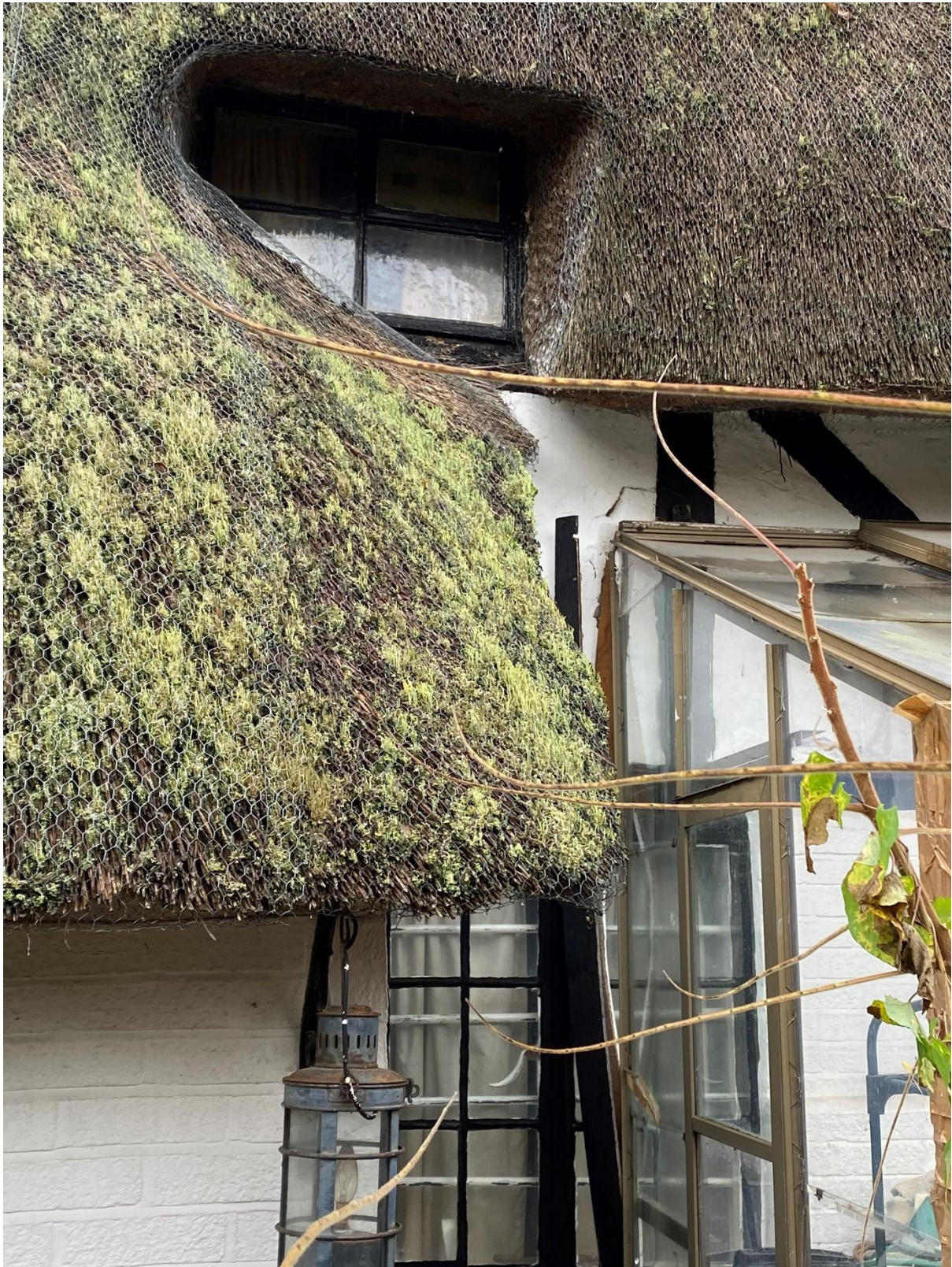
PHOTO 4 – REAR ELEVATION SHOWING HOW THE EXISTING CONSERVATORY DISSECTS THE GF WINDOW
