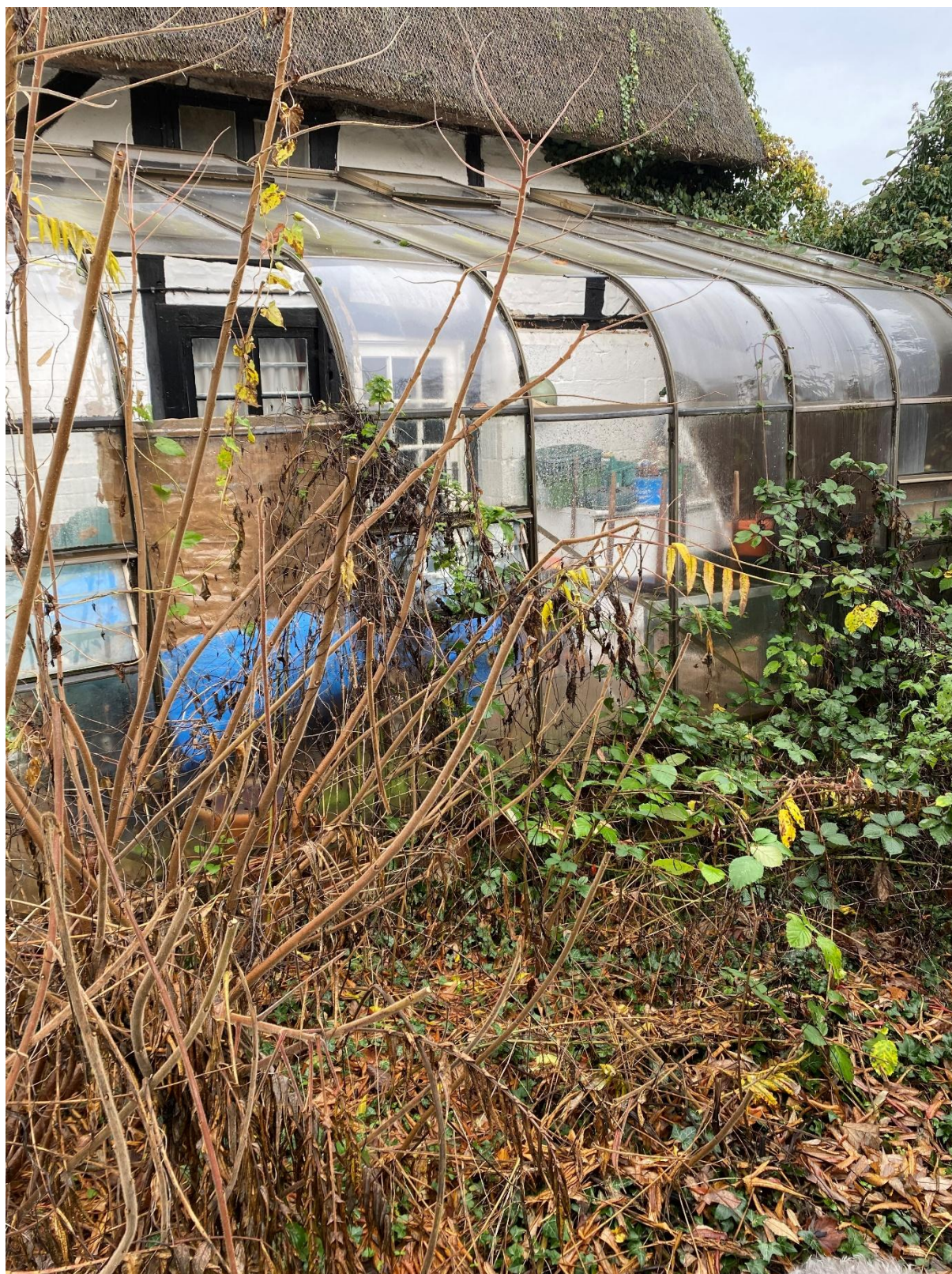
PHOTO 1 – REAR ELEVATION SHOWING EXISTING CONSERVATORY
