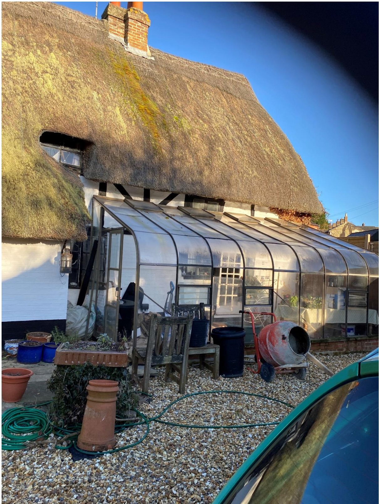
PHOTO 8 – REAR ELEVATION SHOWING HOW THE EXISTING CONSERVATORY SITS ON THE REAR OF THE COTTAGE
