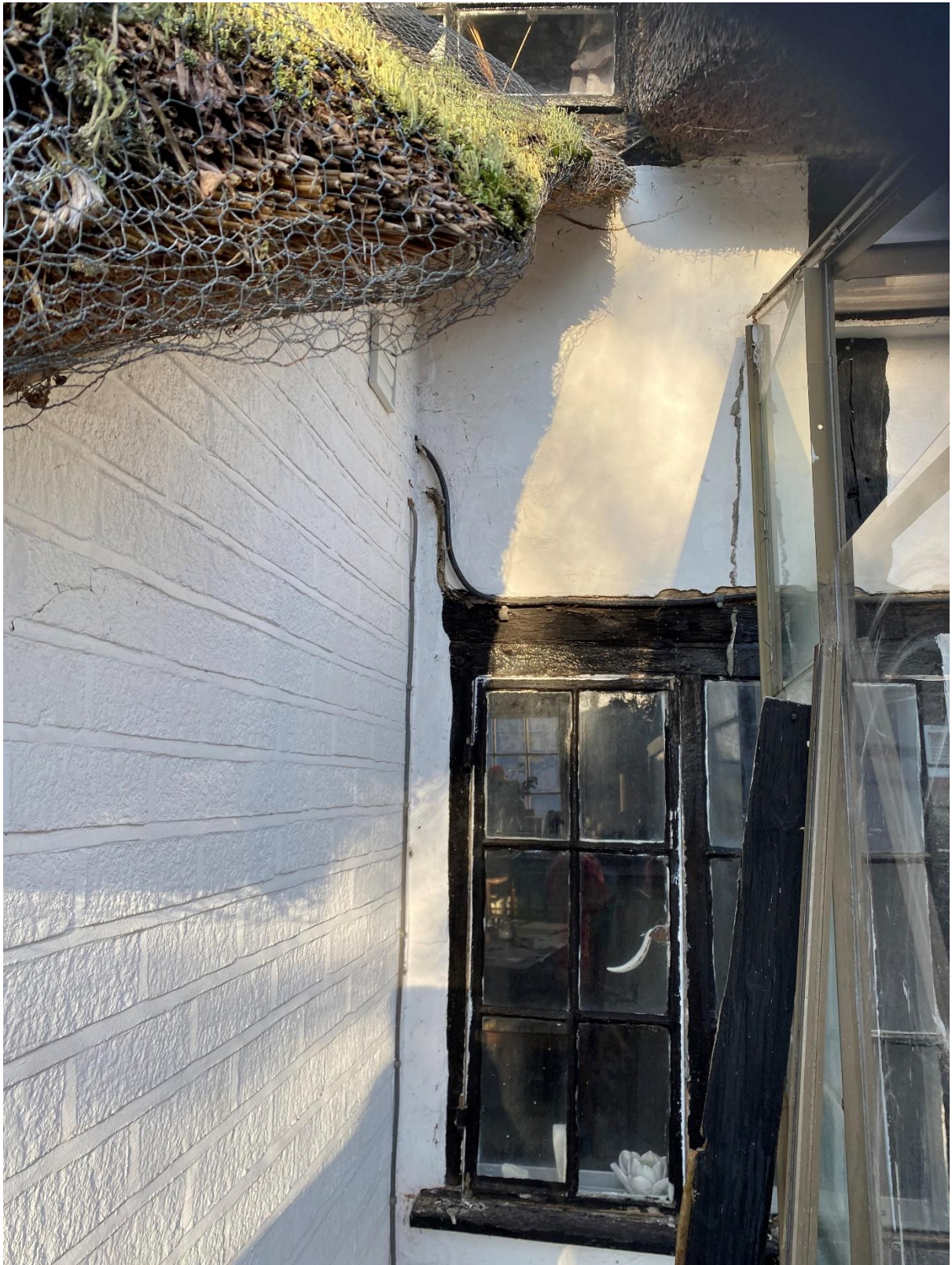
PHOTO 5 – REAR ELEVATION SHOWING HOW THE EXISTING CONSERVATORY DISSECTS THE GF WINDOW
